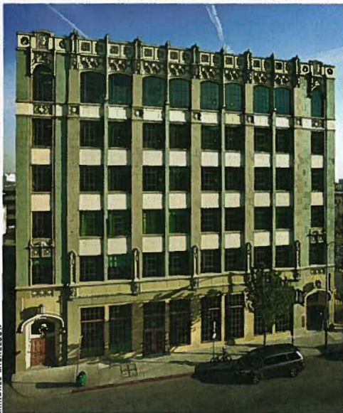
The poured-in-place concrete building not only had its ornamental facade and original windows, but also a few original interior features—in particular, impressive mushroom-cap structural columns and high ceilings. These formed the core for the reuse.
