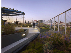
The pavers are pedestal mounted and allow for rainwater to be collected & diverted to an underground cistern.
