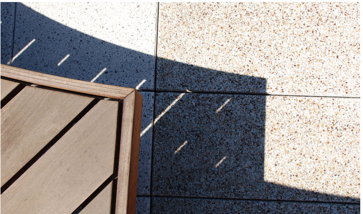
Bench and Paving Detail at Public Roof Garden
