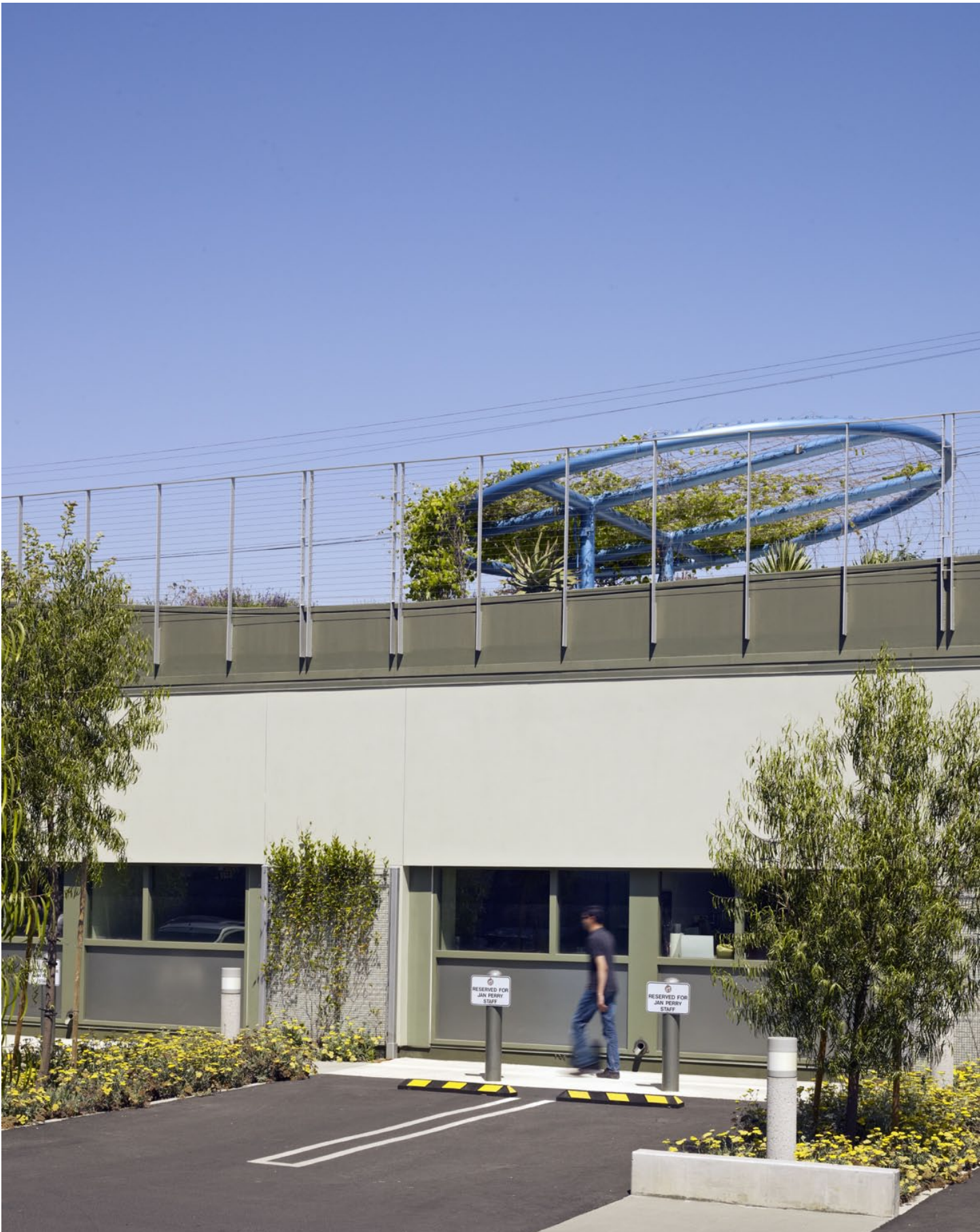
Planted Stormwater Swales in the Parking Lot
