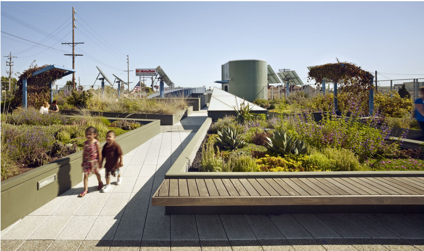
Public Roof Garden
