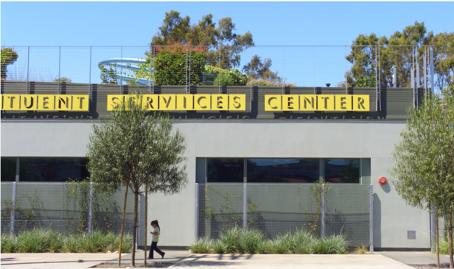
Administration Building and Public Roof Garden from Central Avenue
