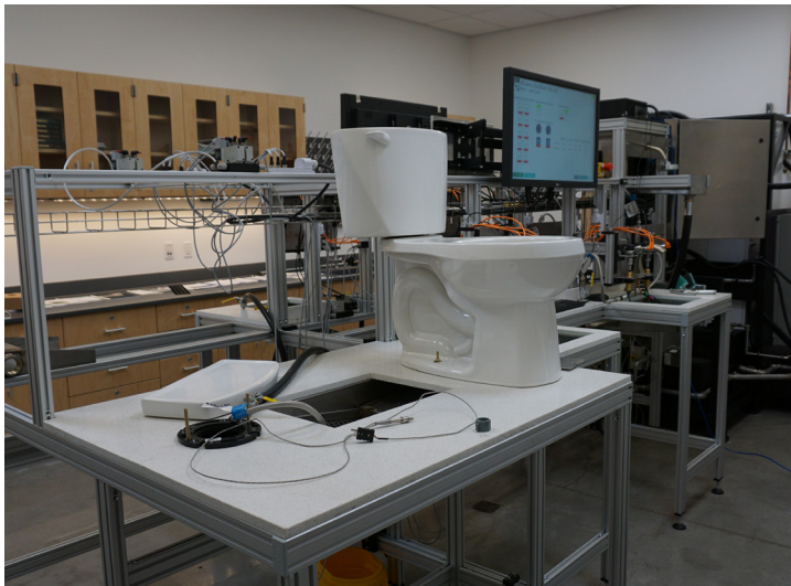
Lighting and plumbing labs allow ESE Group engineers and LACI businesses to evaluate new technology.
