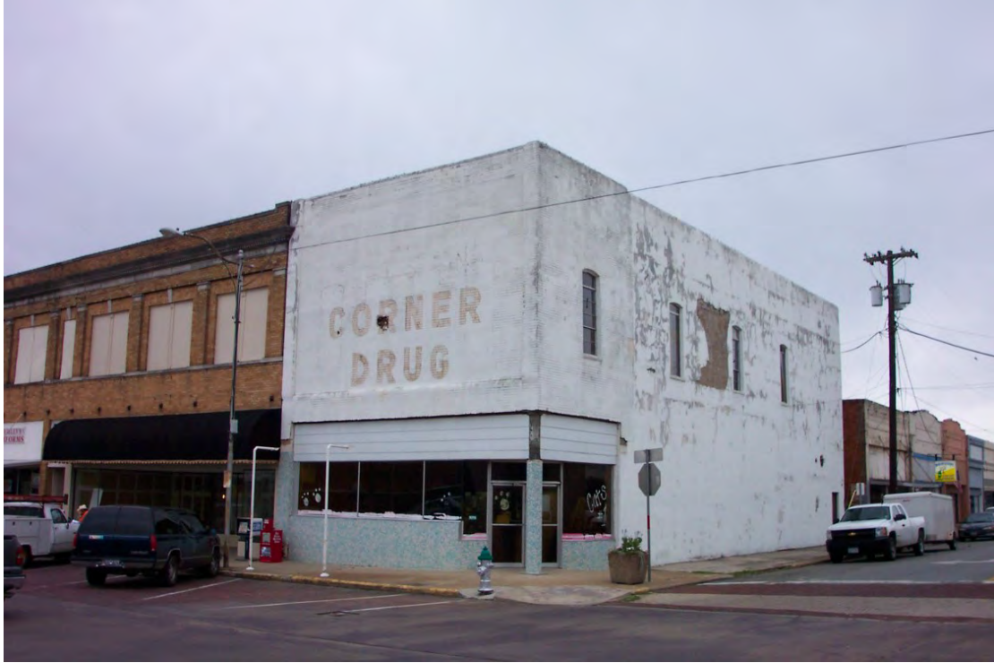
Vacant Building on the Square During the Initial Site Visit
