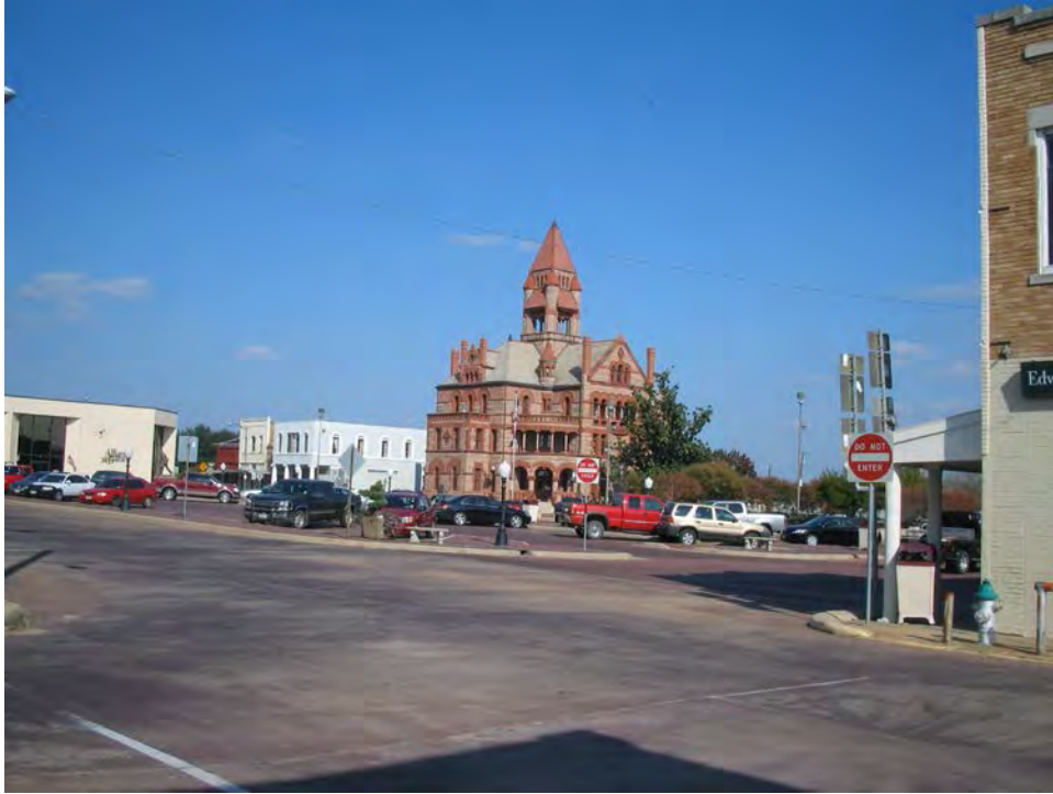
View of the Courthouse Across the Parking Lot (before picture)
