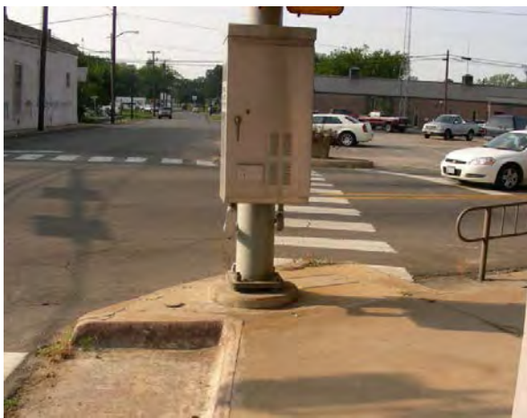
Ugly Signal Pole and Control Box (before picture)
