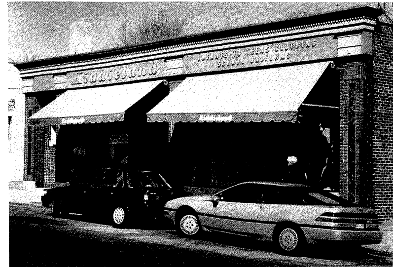
Kiddieland after renovations.
