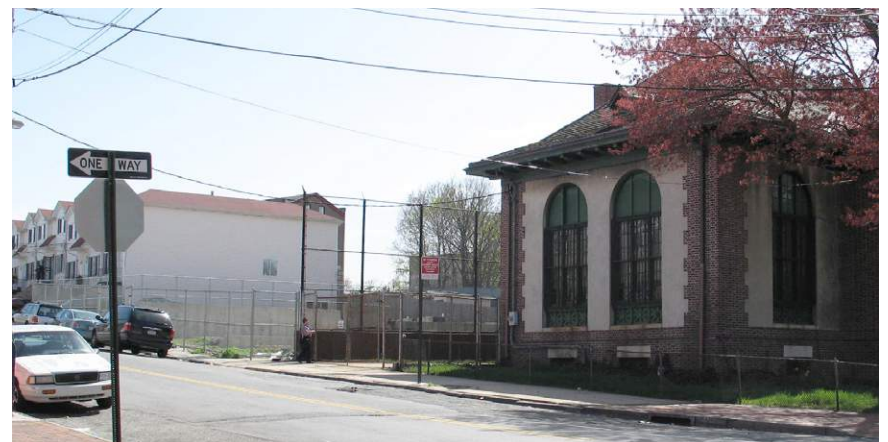
view of library before renovation and expansion
