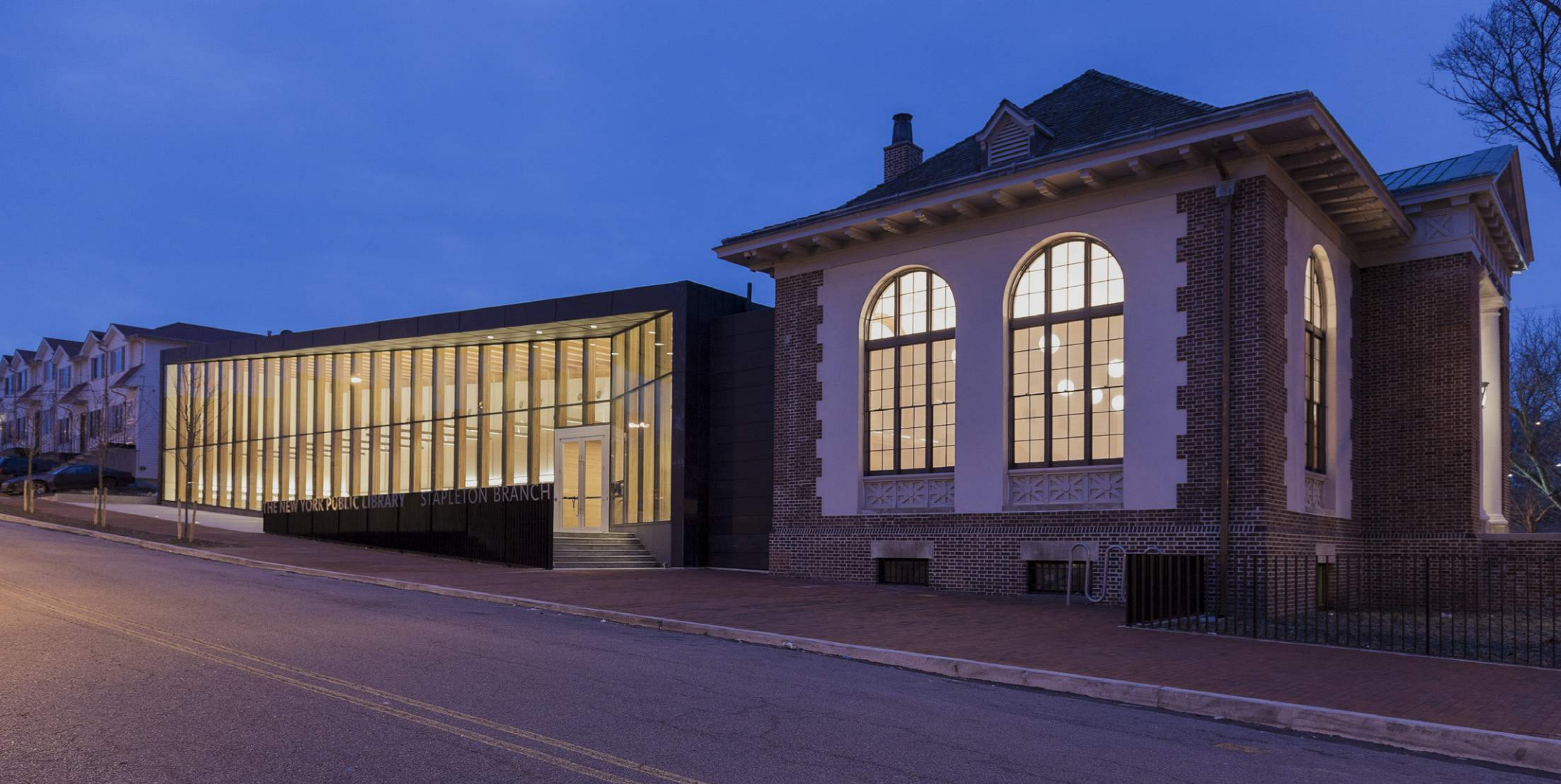
view of entrance from Wright Street looking southwest
