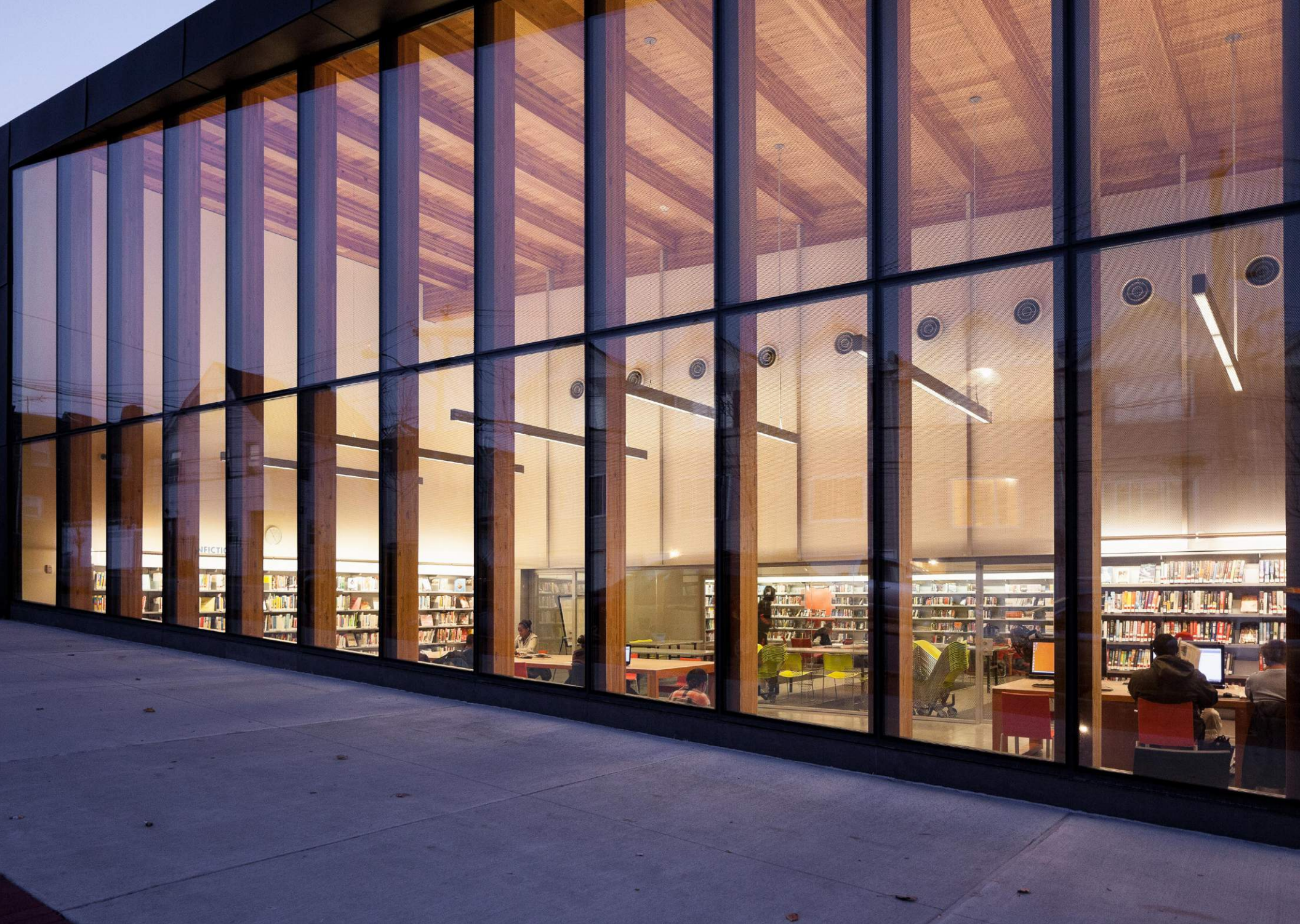
view of the eastern facade and interior at dusk
