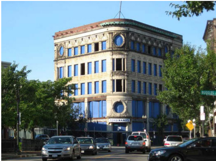
The Bolling Building transformed a vacant building into a highly visible community anchor.
