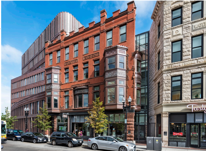
Ground floor storefronts host locally owned businesses that open to the street.
