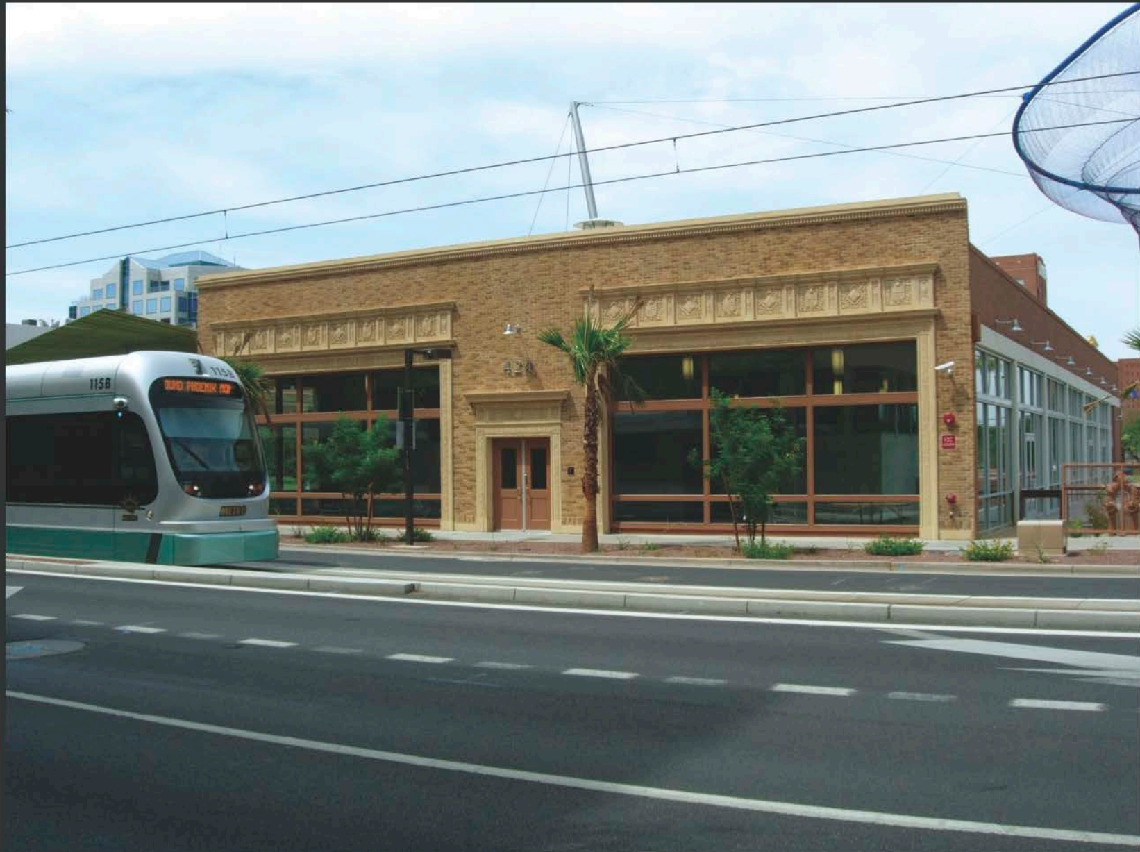
The A.E. England Building, built in 1926 in the Spanish Renaissance Revival style, was adapted for reuse and large windows were restored in reference to its original use as a Hudson and Essex automobile dealership. Inside, the ground-level features restored wood trusses in the exhibition hall and rotating public art exhibitions.
