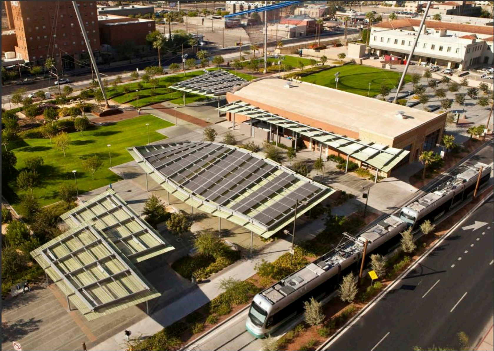
Light Rail trains pass on both sides of Civic Space Park. The undulating shade structures support photovoltaic panels that still allow some light to pass through. The panels produce 75,000 kWh annually, enough to power about 9 homes. Porous concrete, permeable pavers, and decomposed granite are used throughout the site to allow water recharge.
