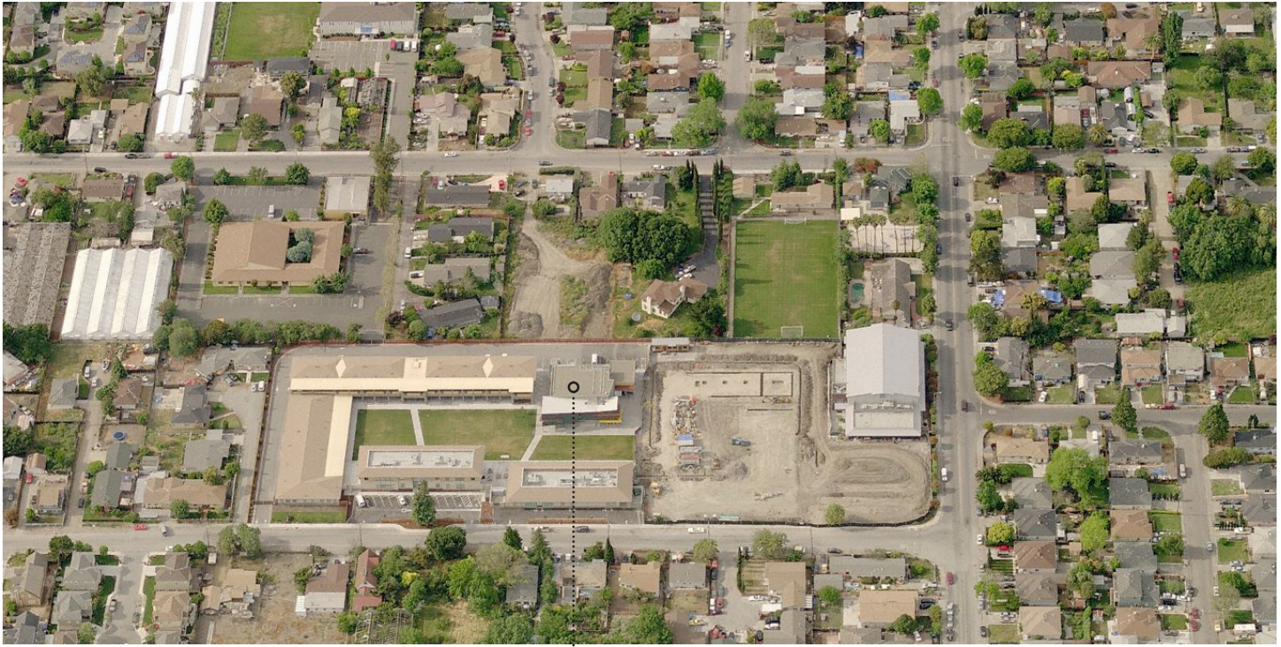
AERIAL VIEW OF CAMPUS UNDER CONSTRUCTION
