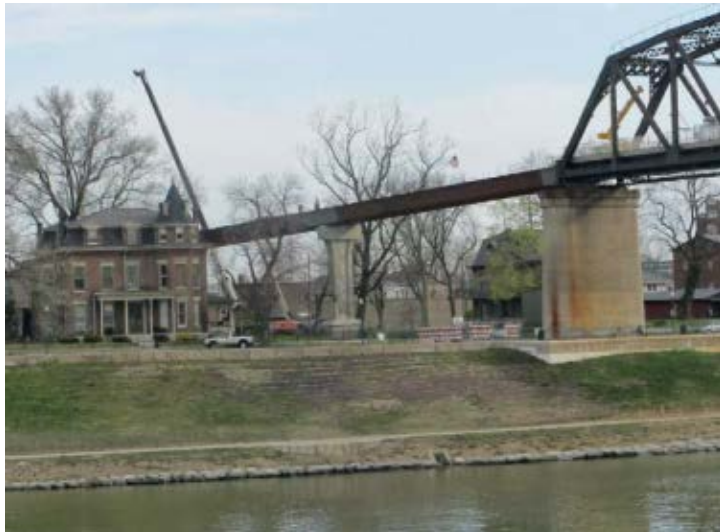
Big Four Bridge Indiana landing under construction
