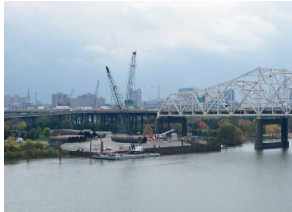
New bridge construction
