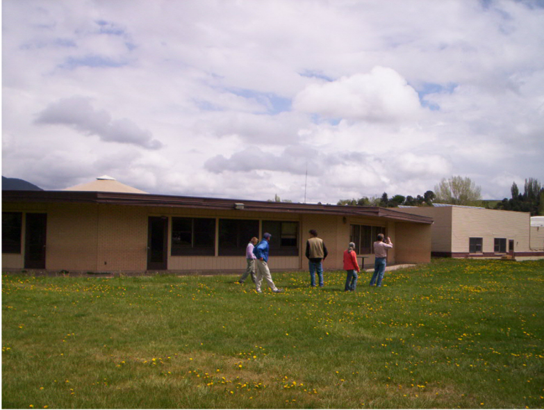
South Exterior Before Renovation
