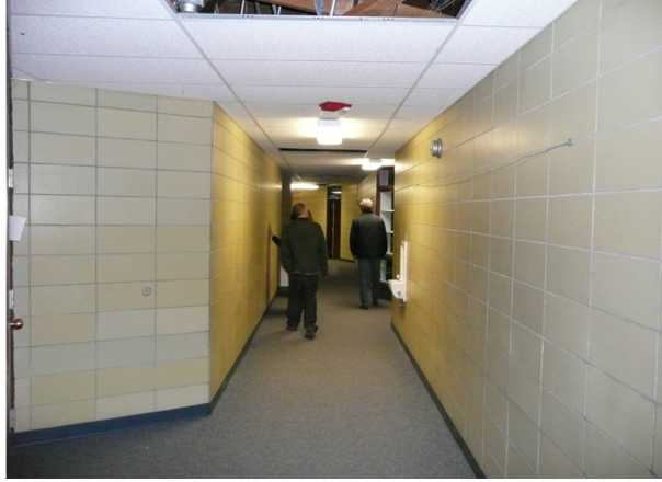
The "Green Mile" Before Renovation
