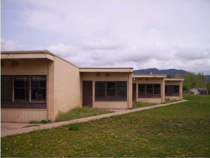
Long Hall Exterior Before Renovation
