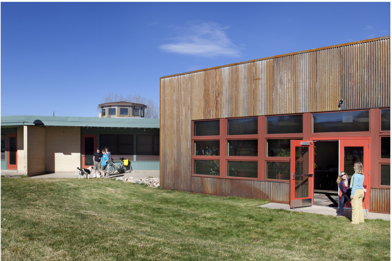
Transformed South Calaway Community Room Exterior
