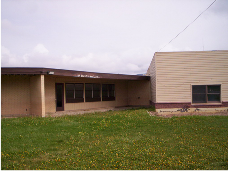
South Exterior Before Renovation
