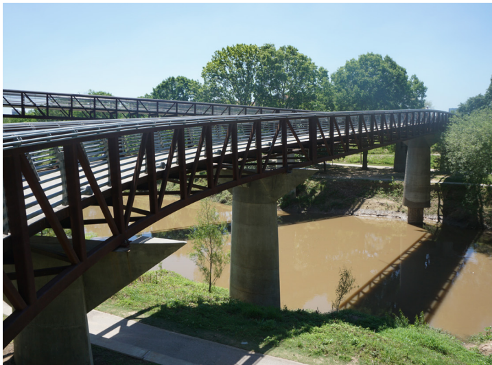
Pedestrian bridges provide access across the bayou.
