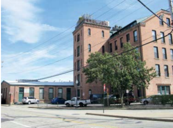
Above: Monohasset Mill; Below: The site prior to remediation
