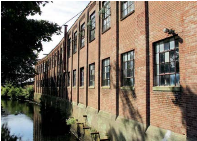
Manufacturing buildings along the Woonasquatucket River
