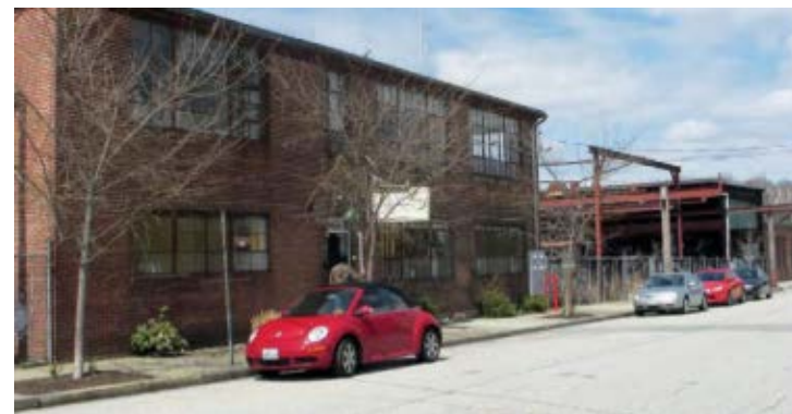
Sims Avenue entrance
