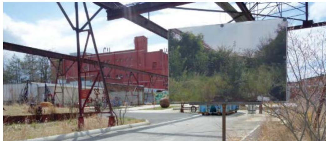
"Before" and "after" views of site
