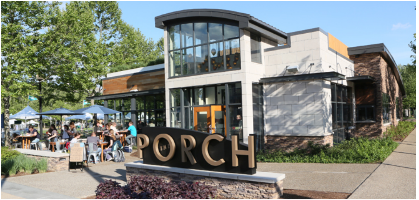
Figure 12 The Porch, the Plaza's Full Service Restaurant
