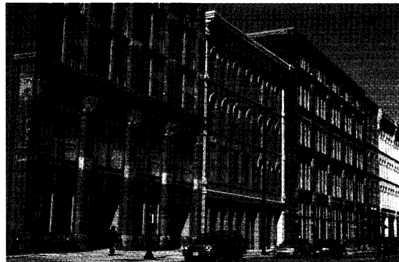
A block of Warehouse District buildings after renovation
