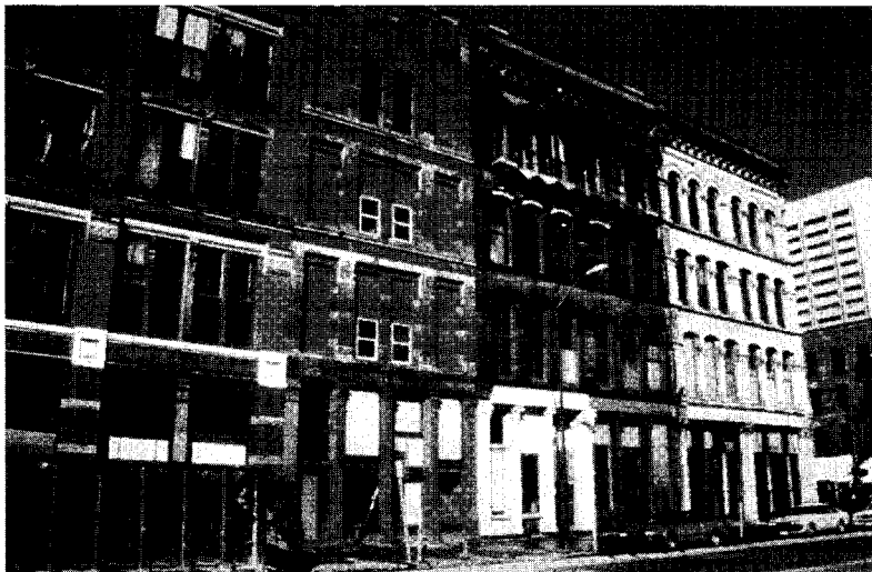
A block of Warehouse District buildings before restoration
