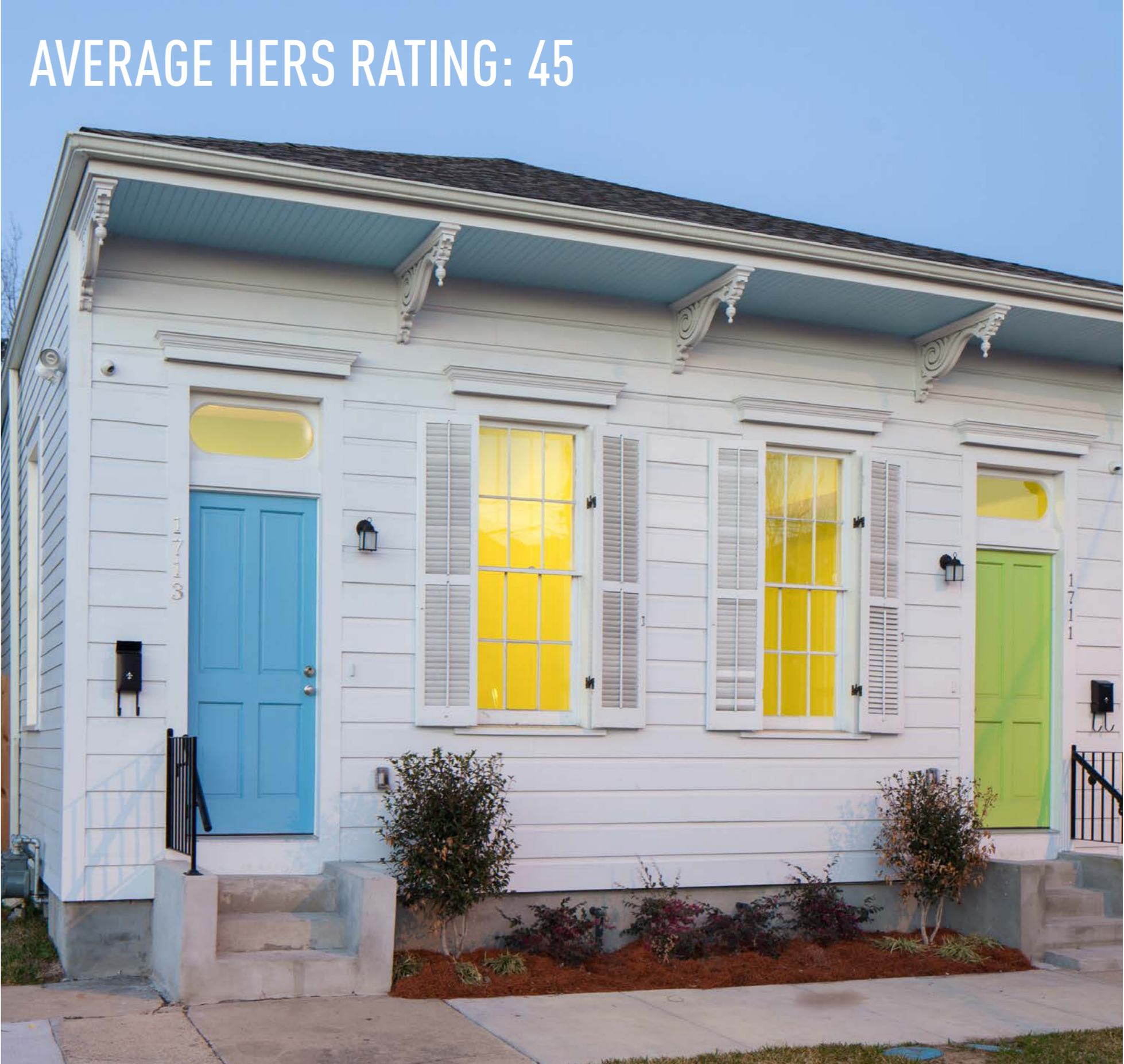
BLOWN CELLULOSE INSULATED RESIDENCE
