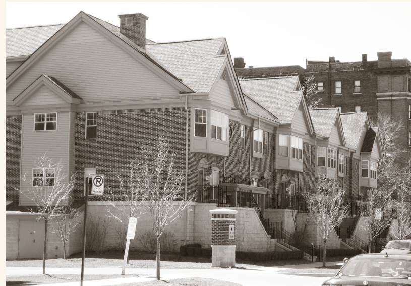
Left: Building being renovated for housing Right: New housing near downtown
