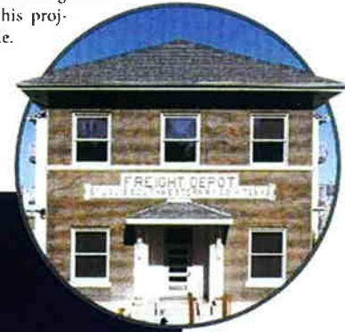
The Depot, Fort Worth
