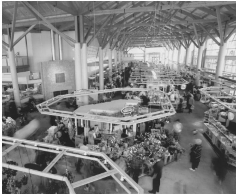
The Market’s L-shaped plan gives it street frontage on three sides with good day-light at all hours.
