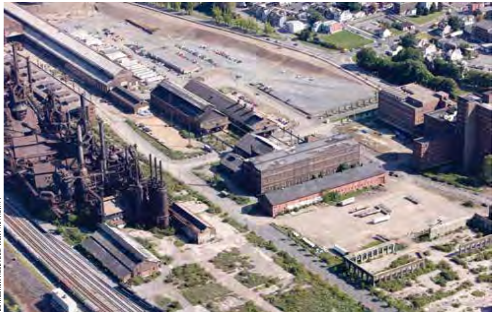
The site before redevelopment.
