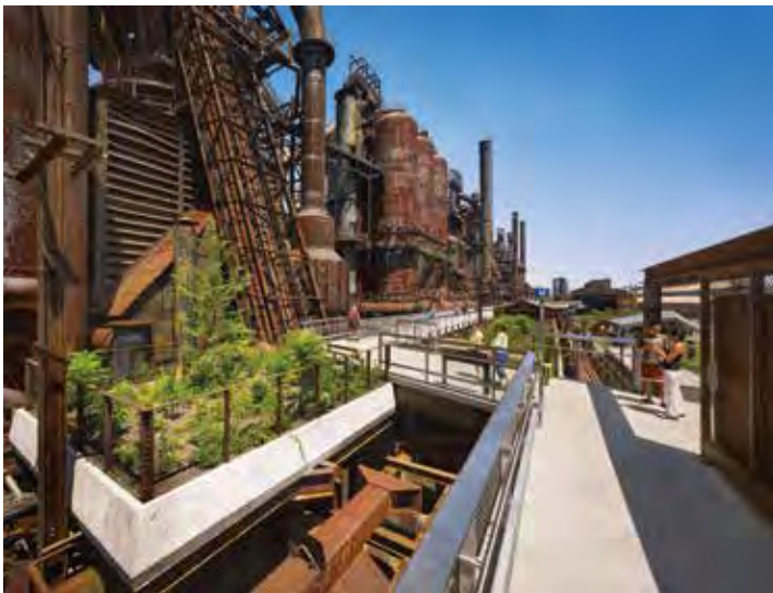
The Hoover-Mason Trestle is a new structure that was placed over and in some places next to the existing rail trestle; the original trestle was used to deliver materials to the blast furnaces.
