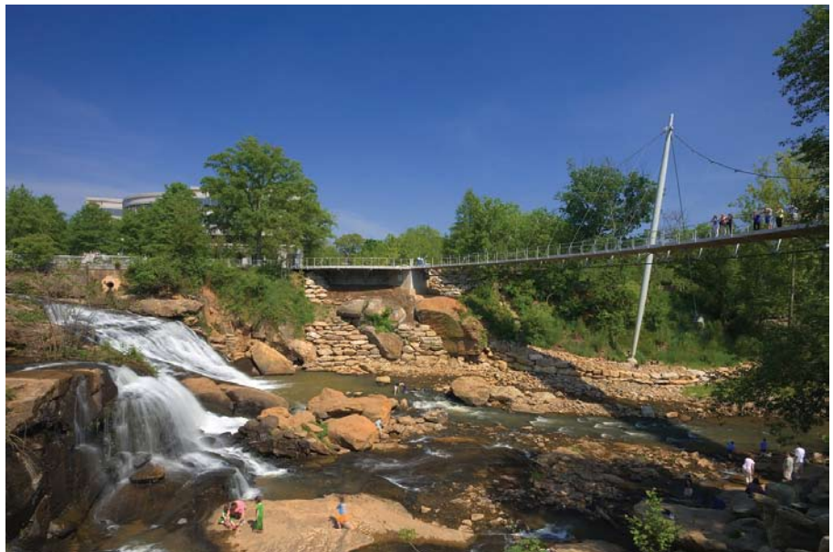
Reedy River Falls is now accessible to visitors and residents alike, making for a water experience unusual in the heart of a city. Photo: Rosales + Partners.
