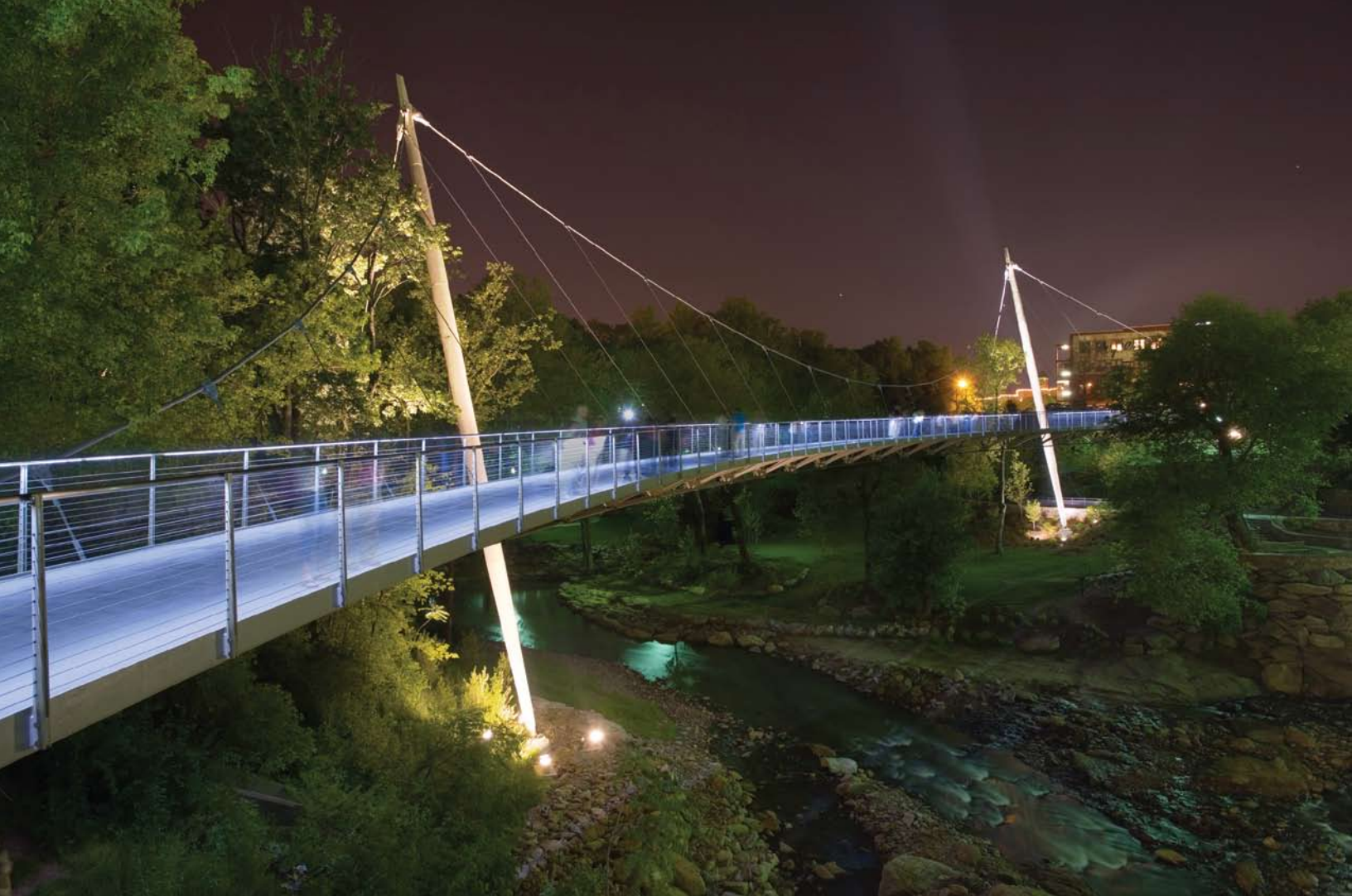
A clear span of 345 feet (105 meters) between the abutments makes the bridge appear to float above the landscape, a dramatic effect accentuated at night by specially designed lighting. Photo: Rosales + Partners.
