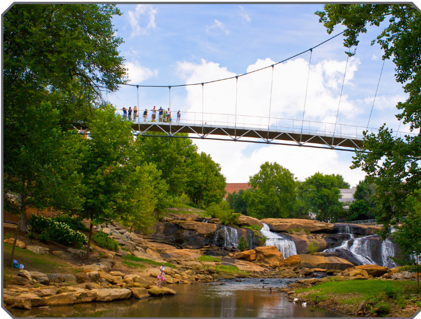
Liberty Bridge, photo credit: City of Greenville
