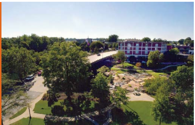
Camperdown Bridge, shown here before its demolition, shaded the waterfall through most of the day so that many Greenville residents were unaware of their city's hidden asset. Photo: City of Greenville.
