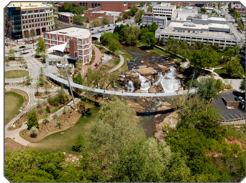
Aerial shot of completed Liberty Bridge, photo credit: Rosales + Partners
