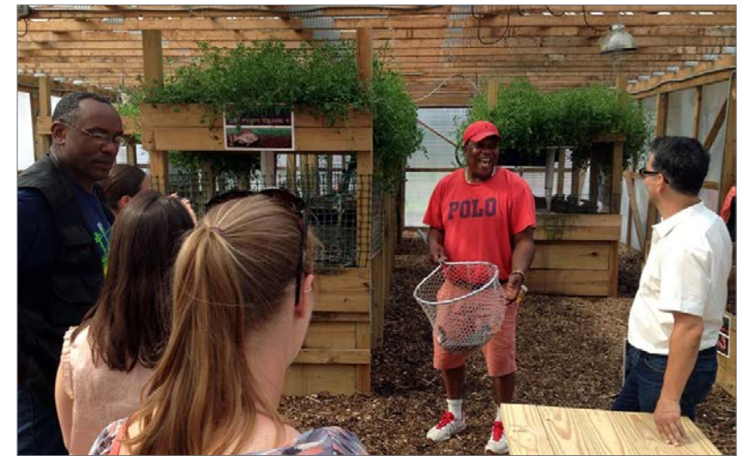
UAIZ Gateway (top): A decorative orchard featuring a twenty-foot-high steel sign that demarcates the Urban Agriculture Innovation Zone is in process on the corner of Kinsman Road and East 81st Street.
