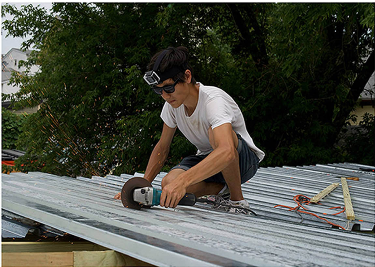
Roof material donated by local roofing company M.Barboza and Sons
