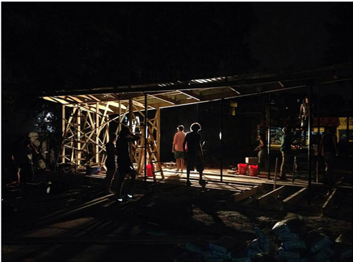
In the last week and a half, construction continued late into the night
