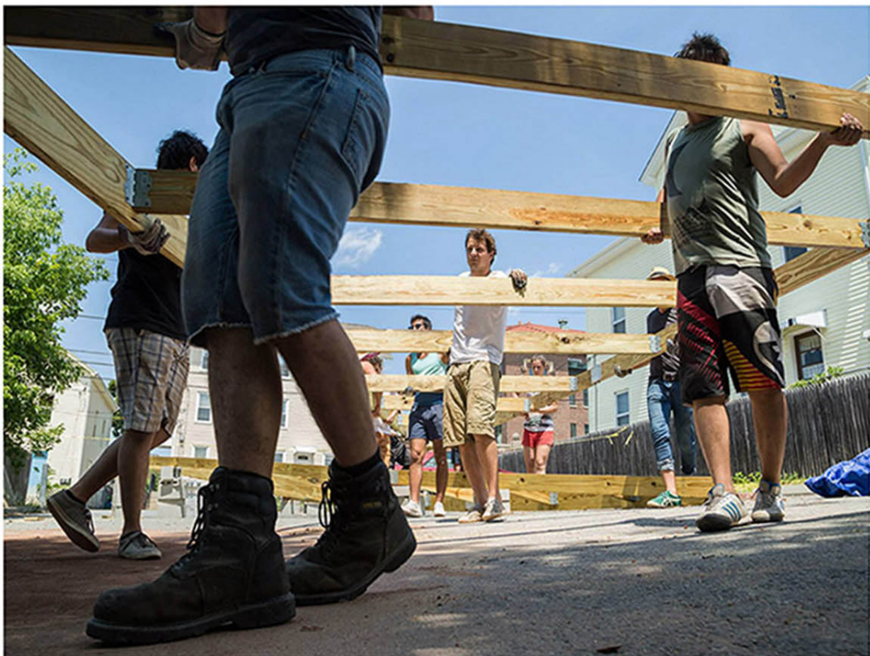
Prefabrication of the roof in adjacent city parking lot
