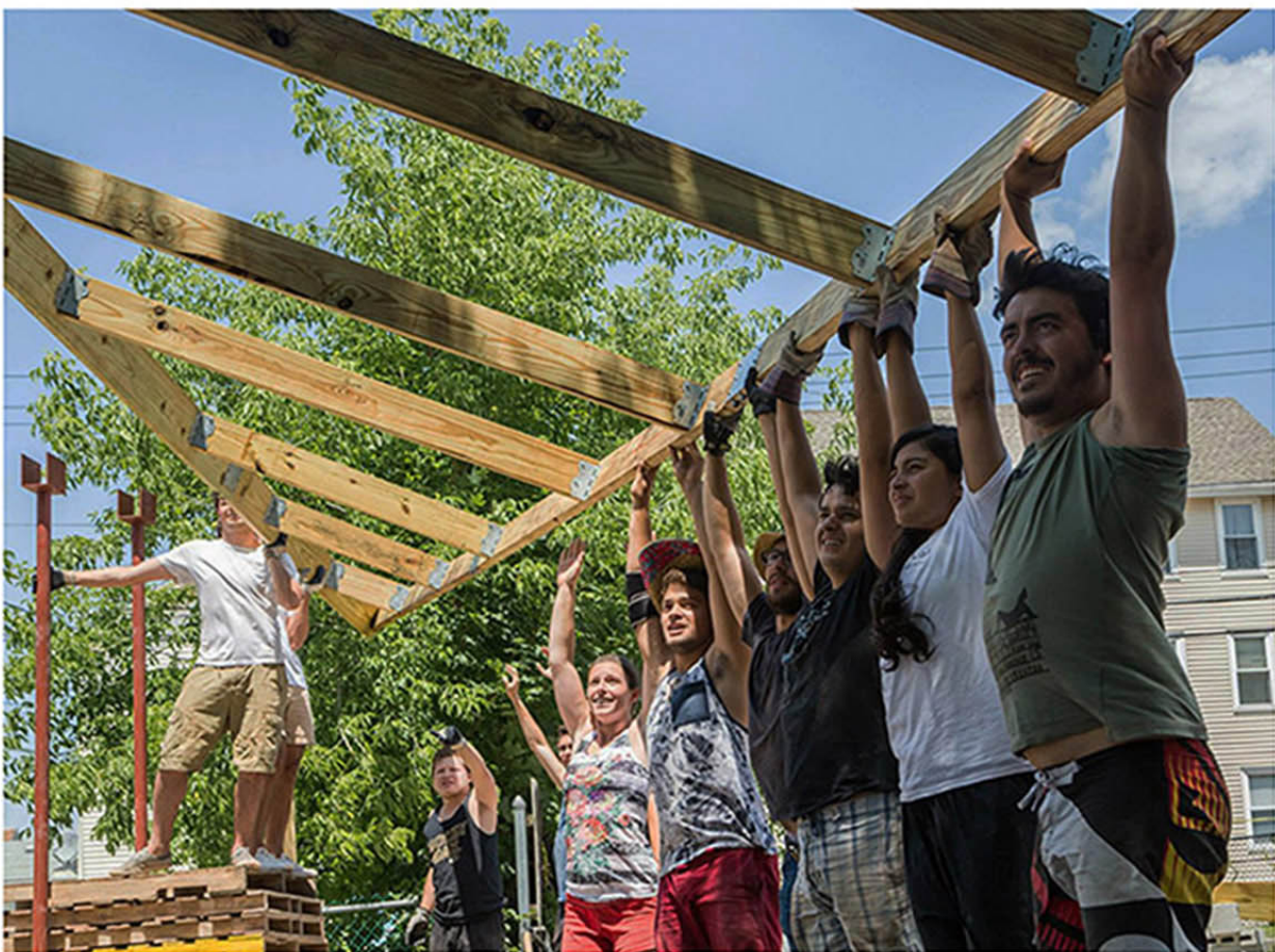
Erecting the roof
