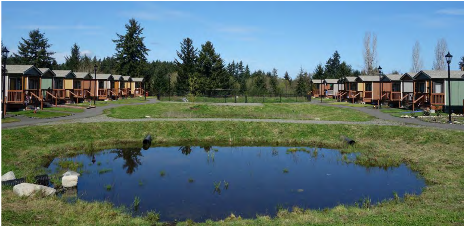
View from community building towards cottages and retention ponds.
