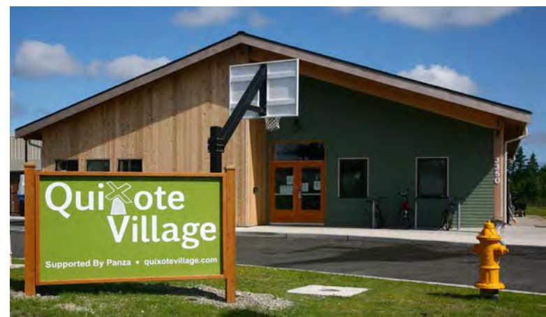
Community building entrance.
