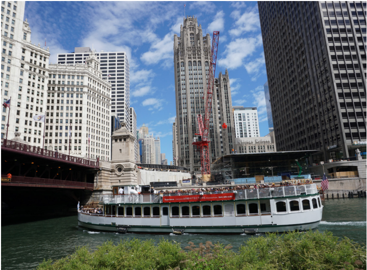
The Riverwalk is attracting new development, including a $27 million Apple store (under construction).
