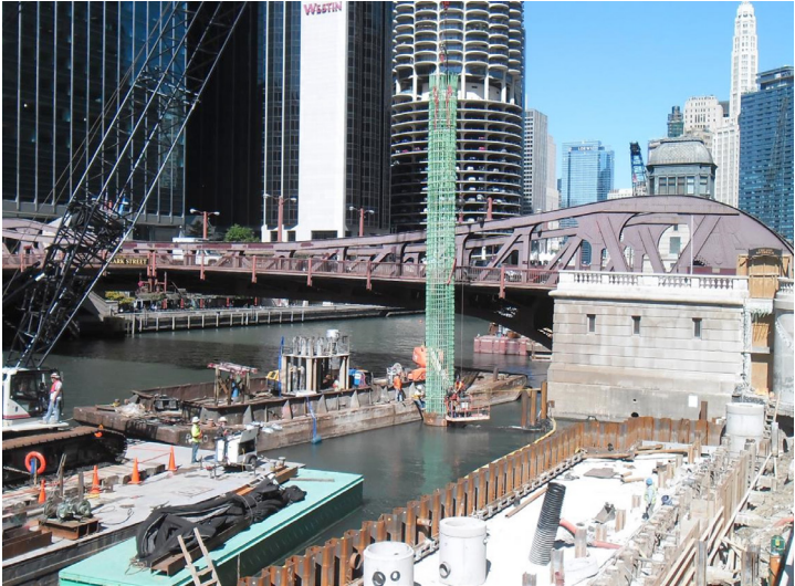
Construction required difficult engineering within complex marine and urban conditions.
