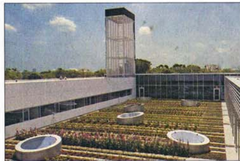
Atop the Comer Youth Center is a courtyardlike roof garden that is directly outside the building's third-floor office. It offers children in the neighborhood a serene place to experience nature. Ronan accented the roof garden with sleek skylights that draw natural light into the building's gymnasium-theater.
