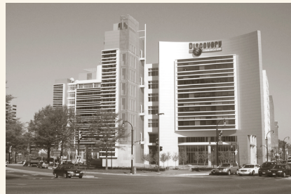
The Discovery Communications Headquarters opened in 2003
