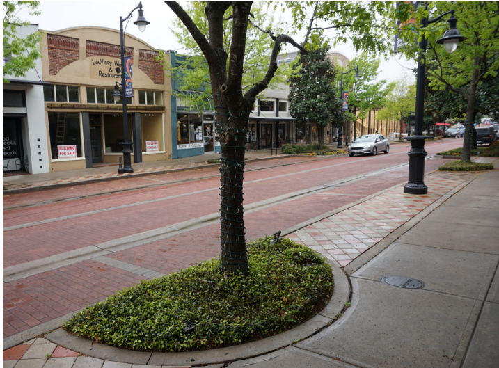
Brick paving, narrow traffic lanes, and parallel parking slow traffic.
