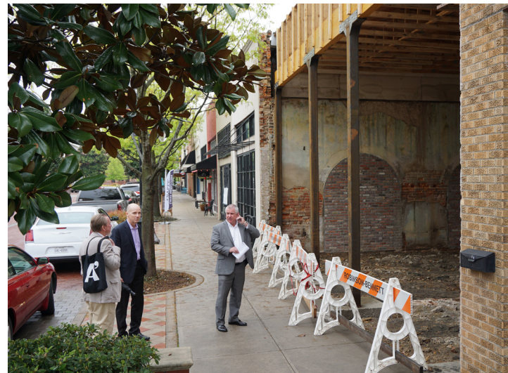
Property owners are improving existing buildings.
