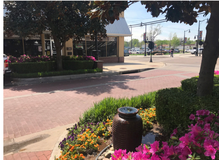
Landscaped “bump-outs” help to capture stormwater runoff.
