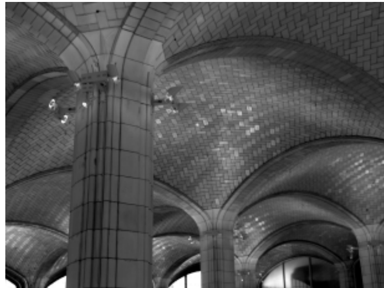
Detail of vaults in Food Emporium
