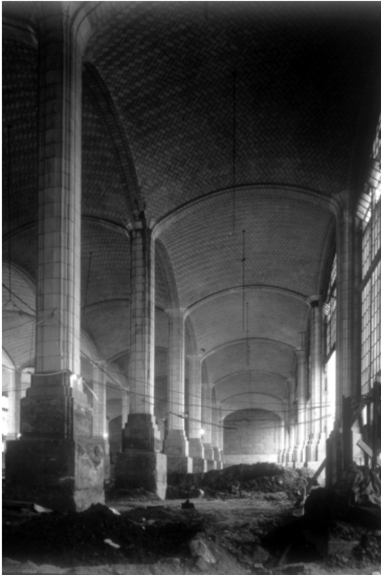
Vaults during construction
