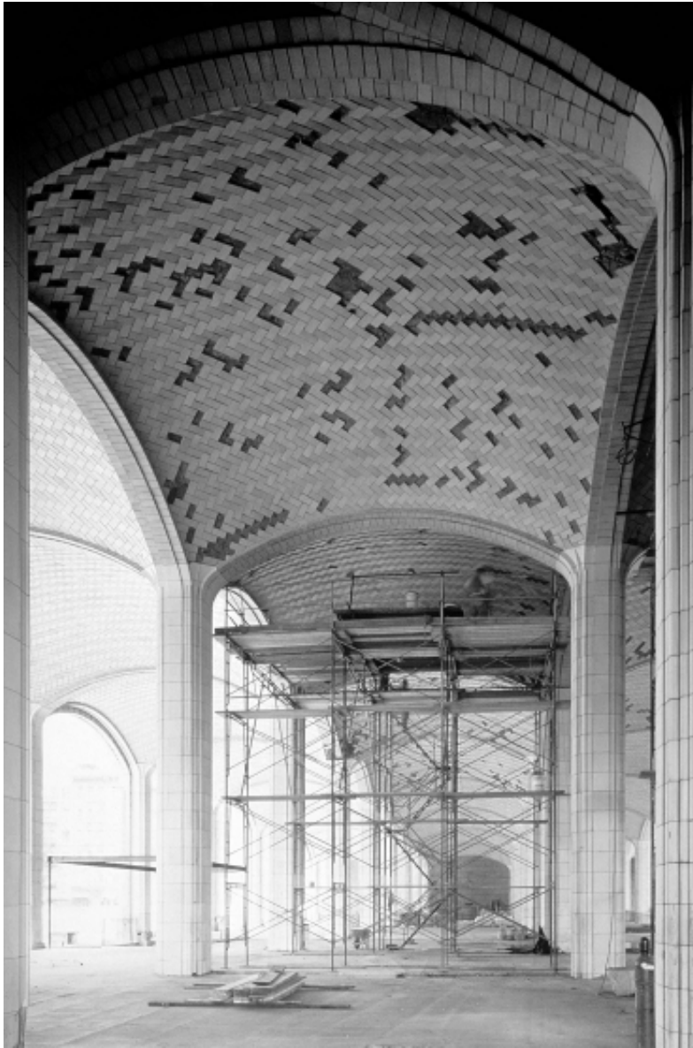
Vaults during restoration
