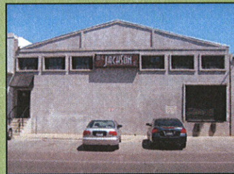
Arizona Hardware Supply prior to rehabilitation, May 2008. Note the non-original, gable-ended roof parapet and stucco sheathing.
