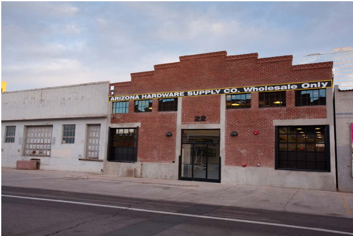
Arizona Hardware Supply Company Warehouse, 22 East Jackson Street
