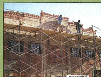
The brick parapet was reconstructed in 2009.
