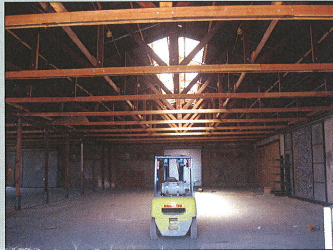
The interior of the Anchor Manufacturing Co. building shows one of the two bays that once housed the iron works and auto body repair shop. An entrance can be seen at center background. The skylight and open doors would have provided the main sources of light when the building was in use.
