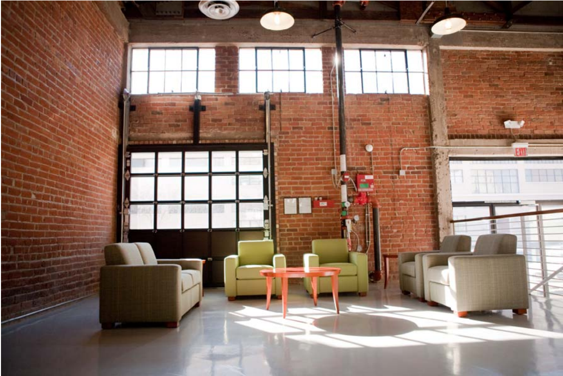
Interior space upon completion. Brick walls and concrete framing are exposed as a key aspect of the interior décor, new doors and windows are in place on ground level. Original restored steel casement sash in upper portion of space were left in place and restored.
