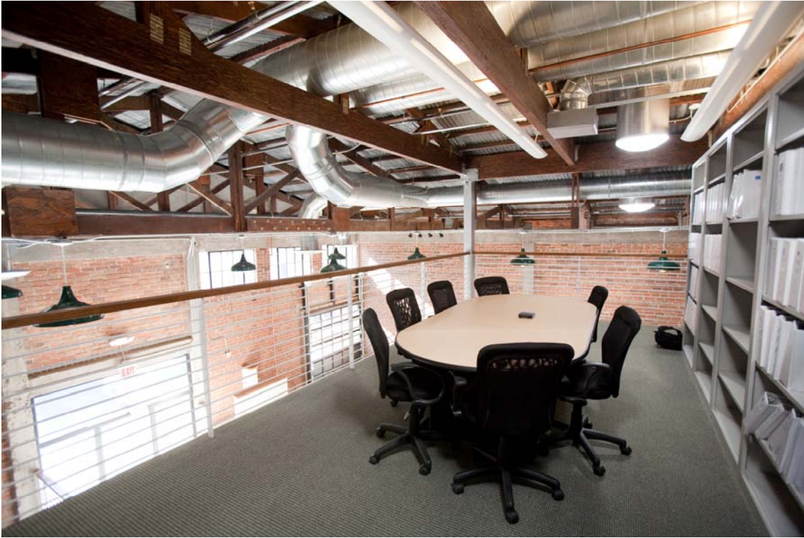
The modification of the roof trusses allowed the mezzanine level to be a “full-height” space for office uses, including offices and conference space.
