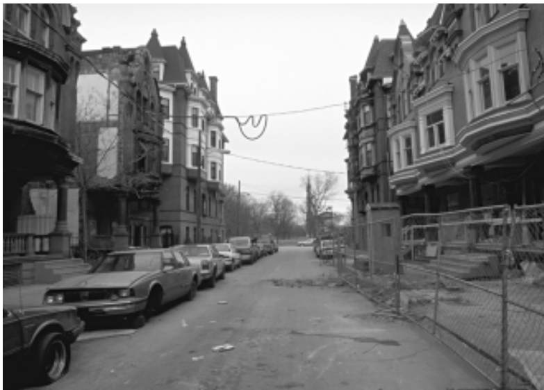
Typical neighborhood street with construction in progress
