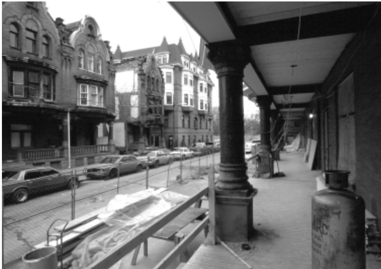
Renovations along Marlton Avenue are in progress
