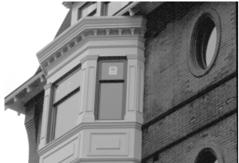
View of the restored Brentwood from Brantwood II, illustrating the simplified molding details on the oval windows.
