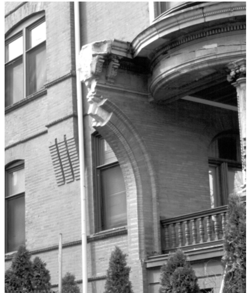
Parkside garden gate detail
