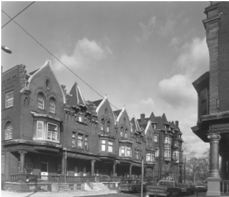
Marlton Apartments under renovation for We Are the People With AIDS/HIV.
