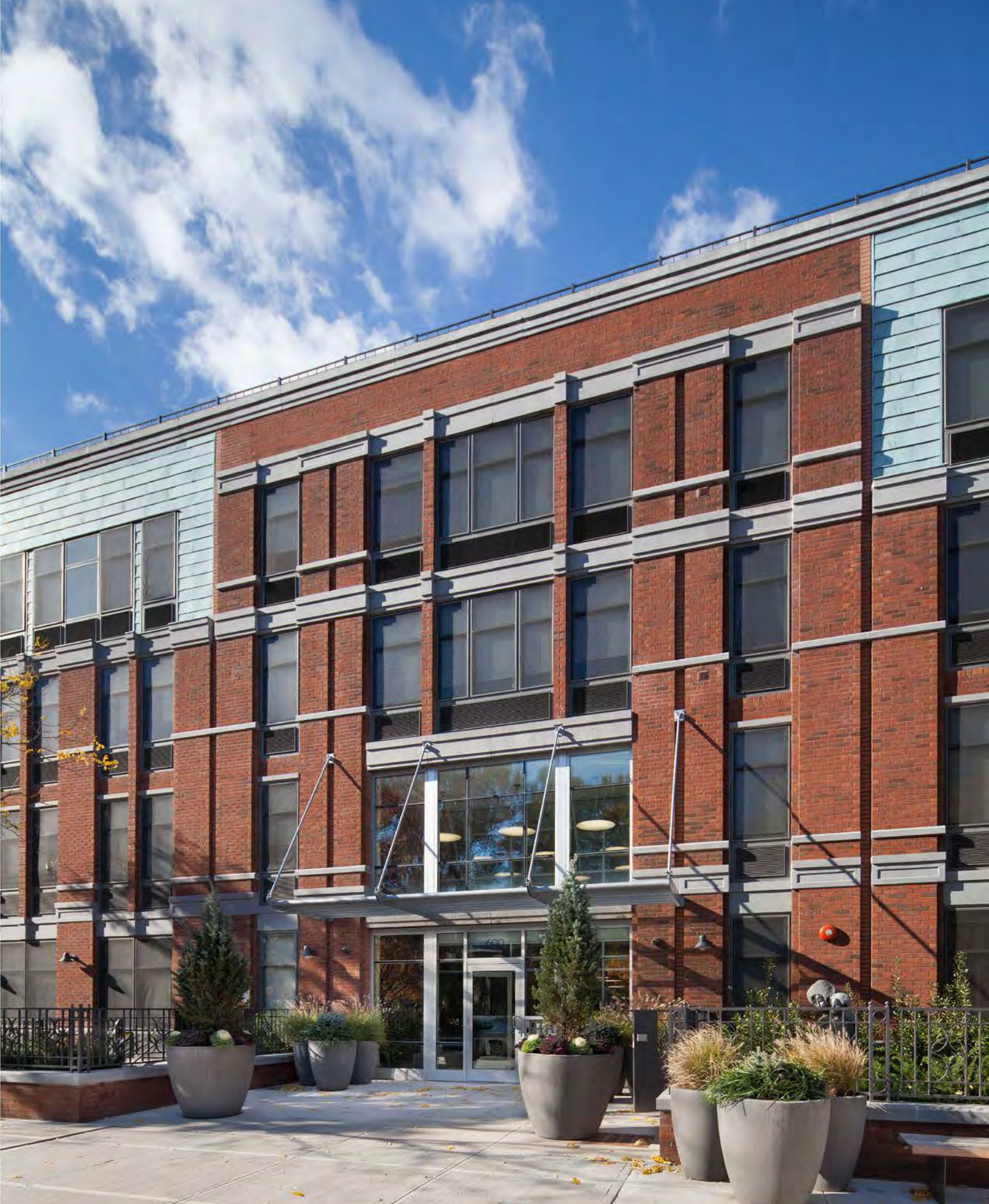
690 ALBANY AVE. MAIN ENTRANCE: Contextual façade materials found in surrounding urban fabric include pre-patinated copper, precast stone edging, and blended red brick. Landscaping provides a softer, welcoming entrance. Two-story lobby curtain wall and metal awning featured in both buildings. Large apartment windows provide ample light. A/C louvers integrated in window assembly.
