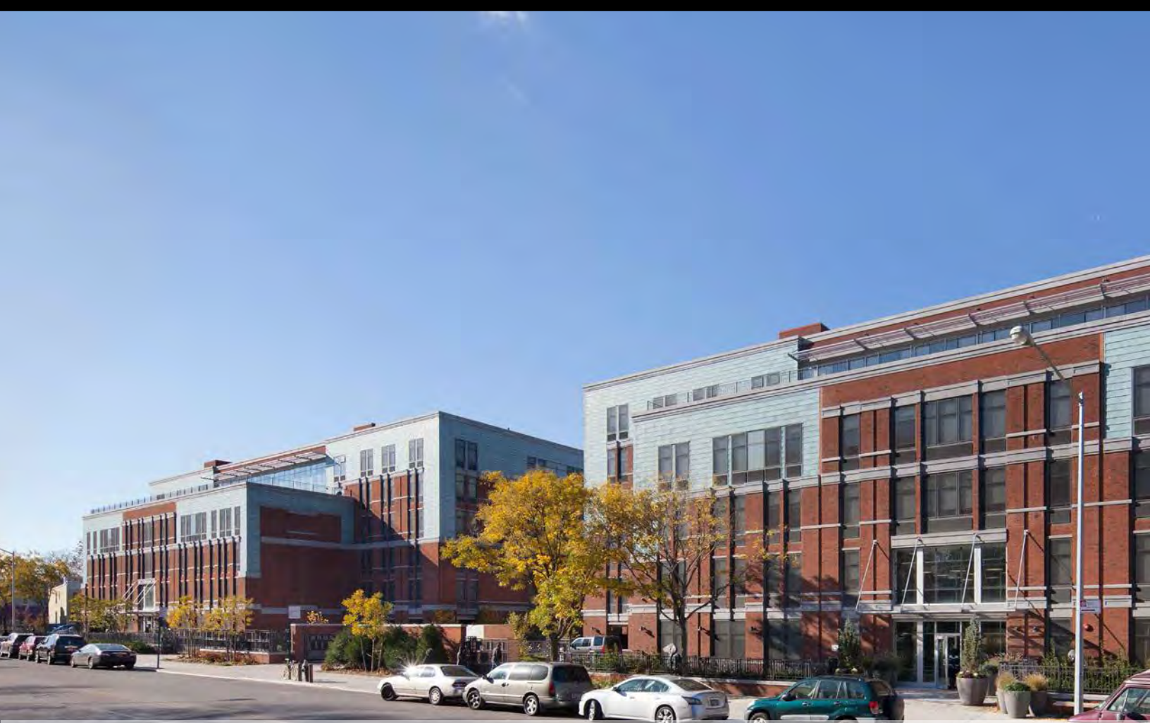
SOUTHERN VIEW (690 ALBANY AVE IN FOREGROUND): Two-story curtain wall allows natural light into lobby and front desk security vestibule, reducing need for electric lighting and energy loads. Streetscape landscaping is designed to provide year-round greenery.
