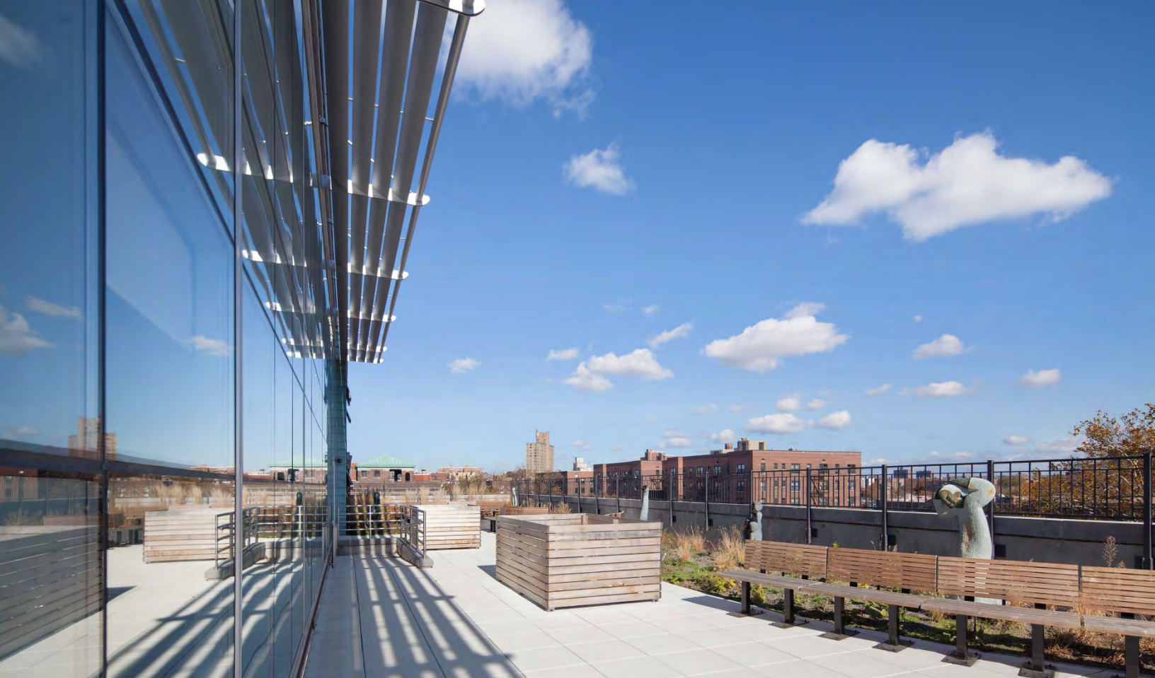
ROOF DECK: Both buildings features an accessible 5 th floor landscaped roof terrace with native plants and unique Zimbabwe sculptures. Custom seating augments tranquil outdoor environment to encourage tenants to occupy the deck. Two-story curtain wall with Brise Soleil allows controlled sunlight throughout 5 th & 6 th floor corridors. Sunshade also provides energy-efficient façade accent.
