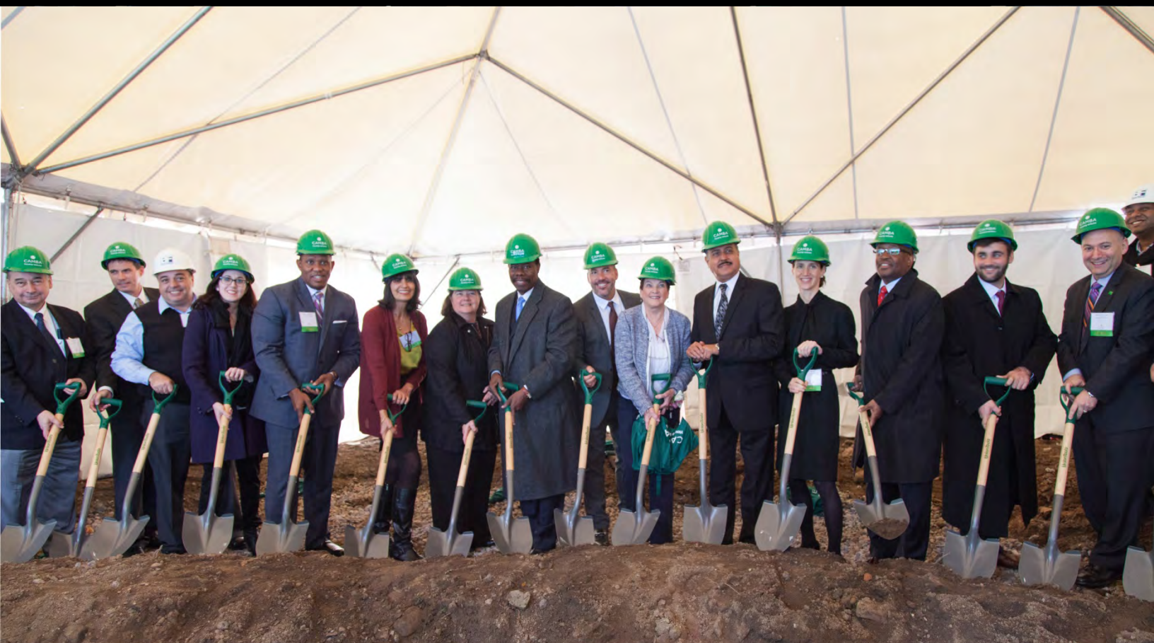
CAMBA GARDENS PHASE II GROUNDBREAKING: The CAMBA Gardens Phase II team celebrated the construction start of Phase II. By closing on CGII, CHV successfully replicated the national model of developing sustainable, affordable and supportive housing on underutilized public hospital land, thereby providing tenants with access to neighboring medical services.
