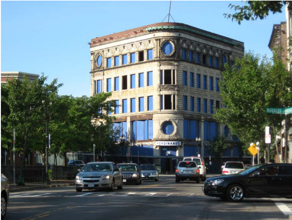
Existing conditions view of Ferdinand Building
