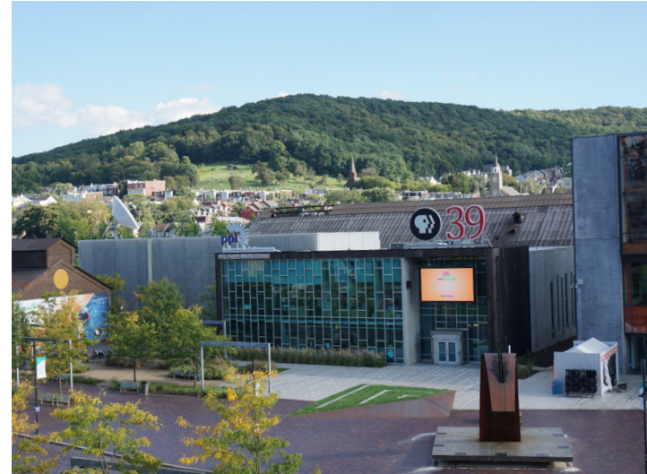
PPL Public Media Center at PBS 39 houses the local public broadcasting station.
