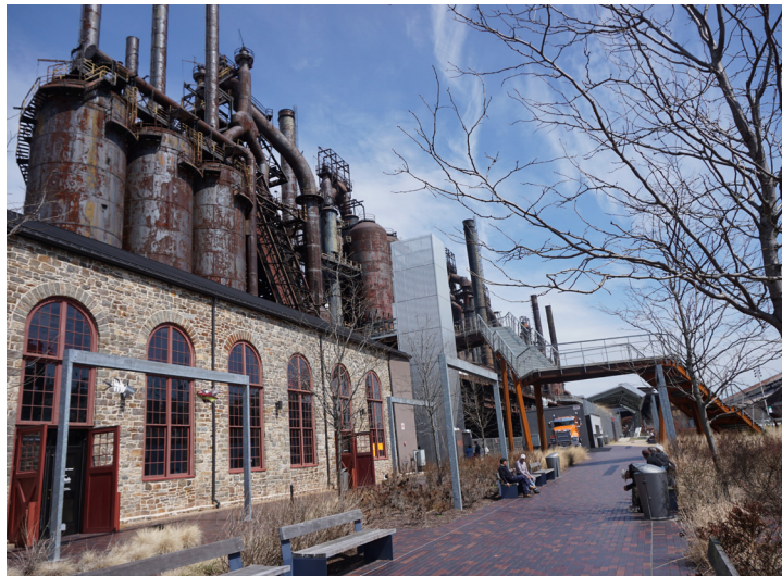
The stone Stock House was renovated into the Bethlehem Visitor Center.
