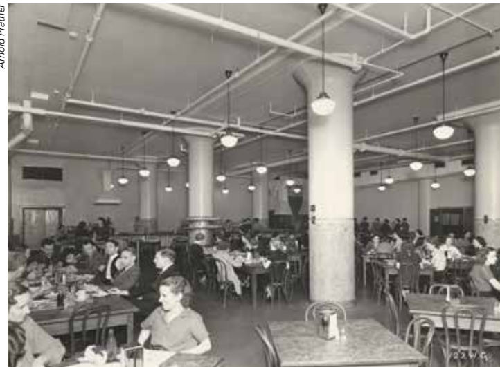
The building followed a standardized design that used a grid of reinforced concrete piers.
