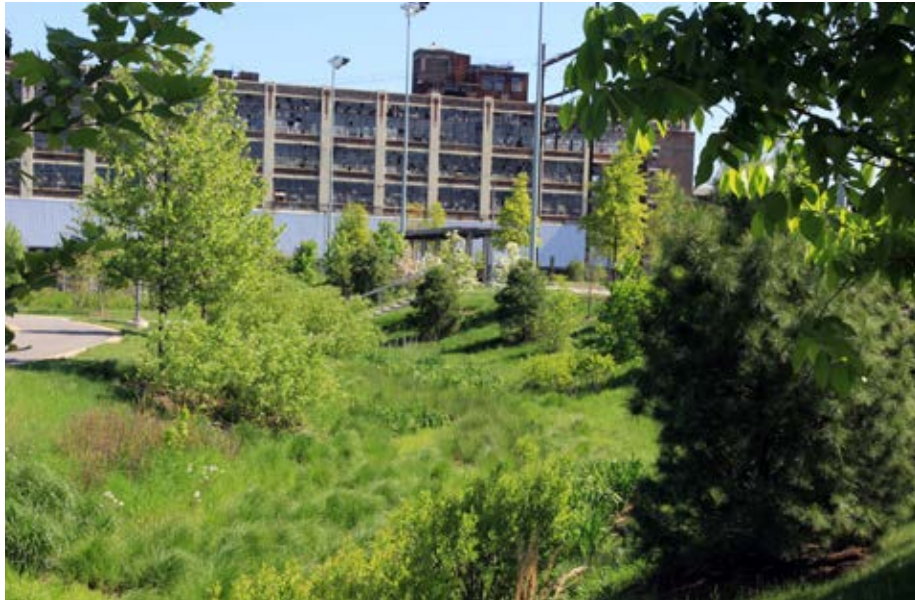
Figure 7 Rain gardens behind the building are located to take advantage of the gradient of the former rail spur. Slope on the right is fed by storm water infiltrated from the recreation field. (photo by K.Daryl Carrington, May)
