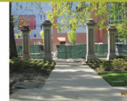
SALVAGED & RENOVATED COLUMNS
