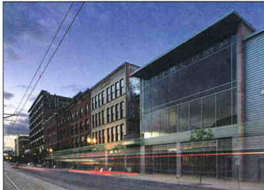
From Left, The Harmon, McDonald & Smith and Cherry Parkes buildings and Philip Hall, seen from Pacific Avenue
