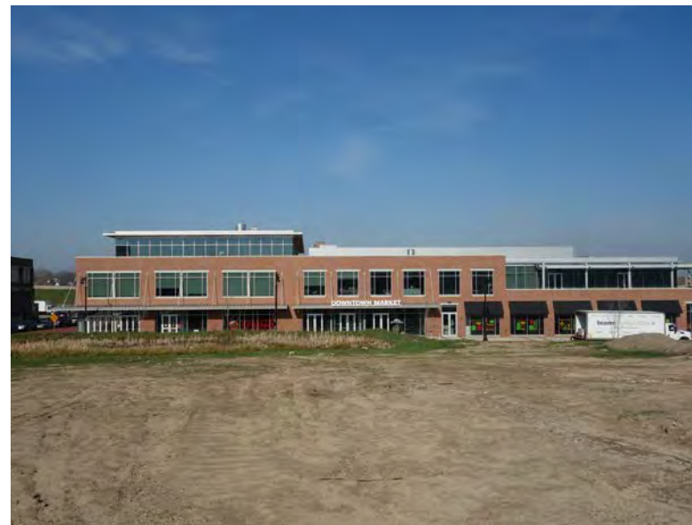
Views of the Ionia Avenue facade.
