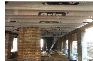
SPRAY FOAM INSULATION
