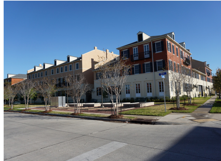
The Lafitte public housing project has been redeveloped into the new mixed-income community of Faubourg Lafitte.
