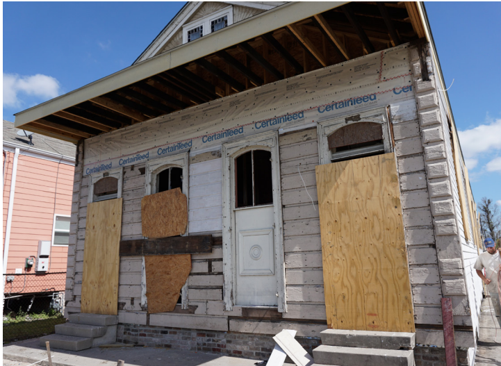
Original architectural details like wood windows, exterior siding, and brackets were preserved.
