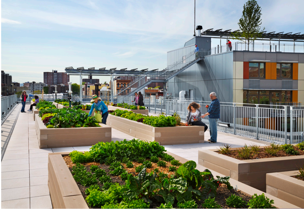
10. Fifth Floor Garden Roof Looking North/Vegetation
