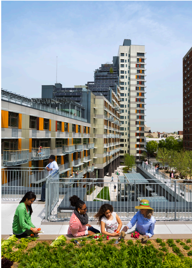
8. Fifth Floor Garden Roof Looking North
