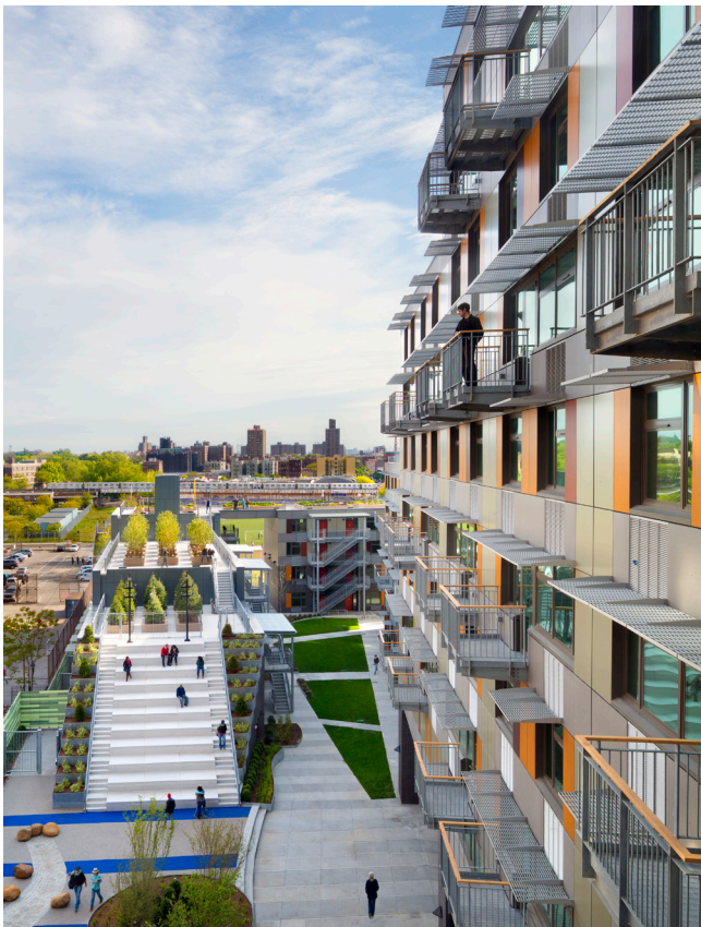
6. Courtyard Facade Looking South
