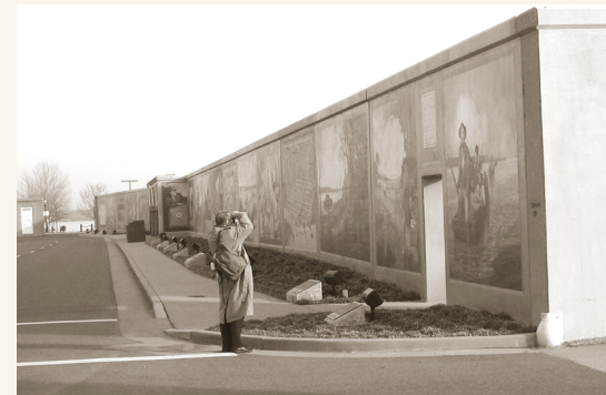
Flood control barrier on the Ohio river
