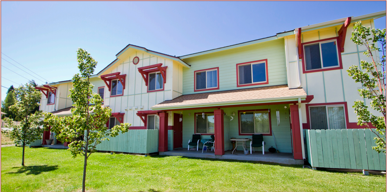
2 of 13 Three-Bedroom townhomes – back view
