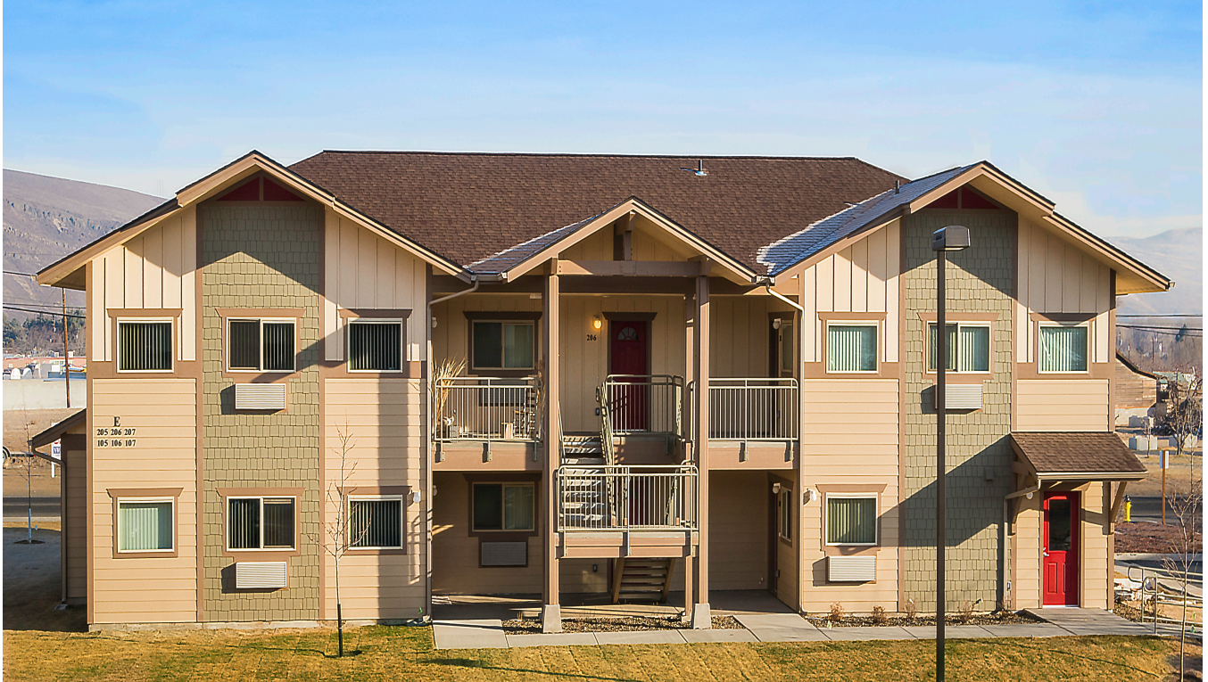
One of four six-plexes in Phase III
