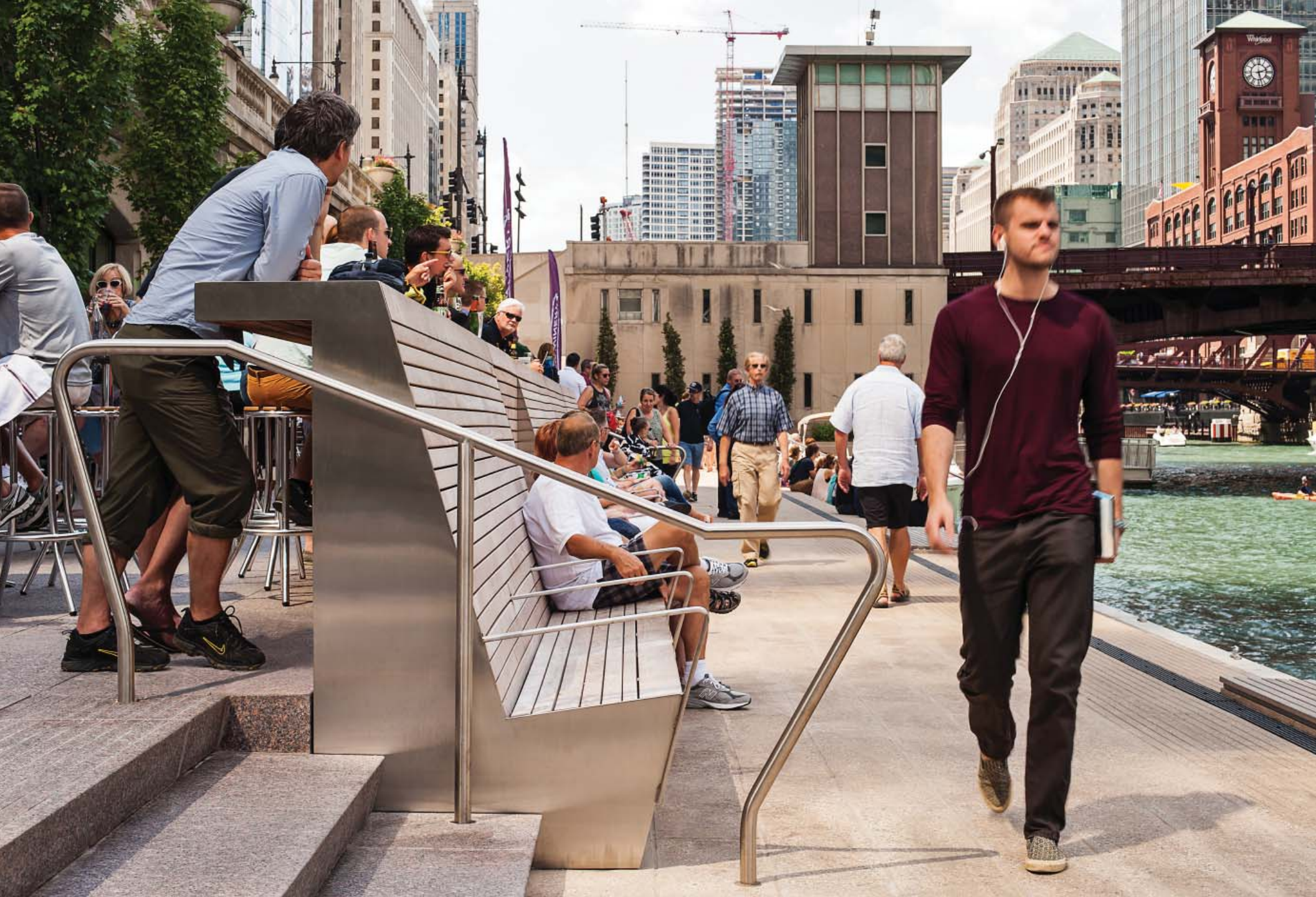
The project's material language takes its cues from the adjacent architecture. The upper section matches the limestone and granite of the Wacker Drive Viaduct and Bridgehouses. The lower (flood prone) section is more rugged precast concrete and metal like the hulking bascule bridges.
