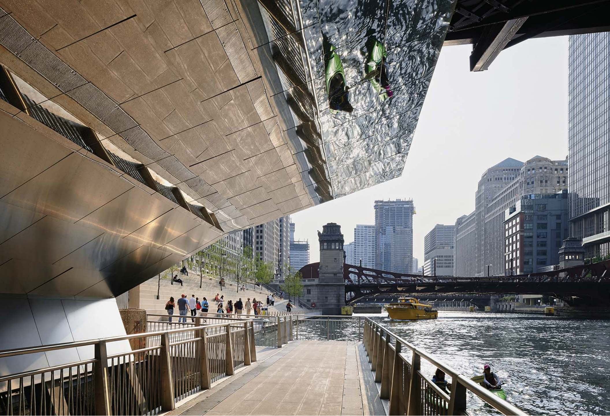
A series of "underbridge" crossings connect blocks that had been previously discrete spaces. These stainless steel-canopied mini-bridges both shelter pedestrians as they pass beneath the bridge deck above and reflect the texture and light of the river's surface.
