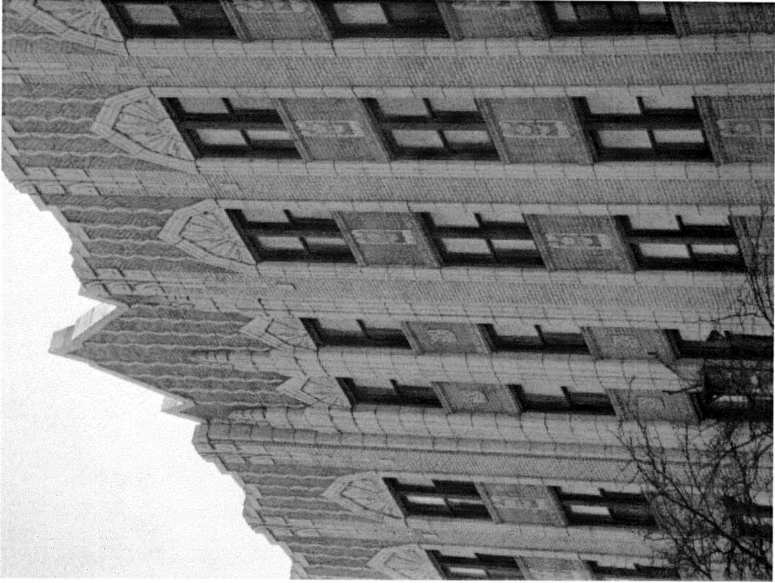
Above: The combination of the continuous vertical piers with the understated spandrel panels lends the Union Park Hotel a strong vertical emphasis, another important trait of the Art Deco style.
