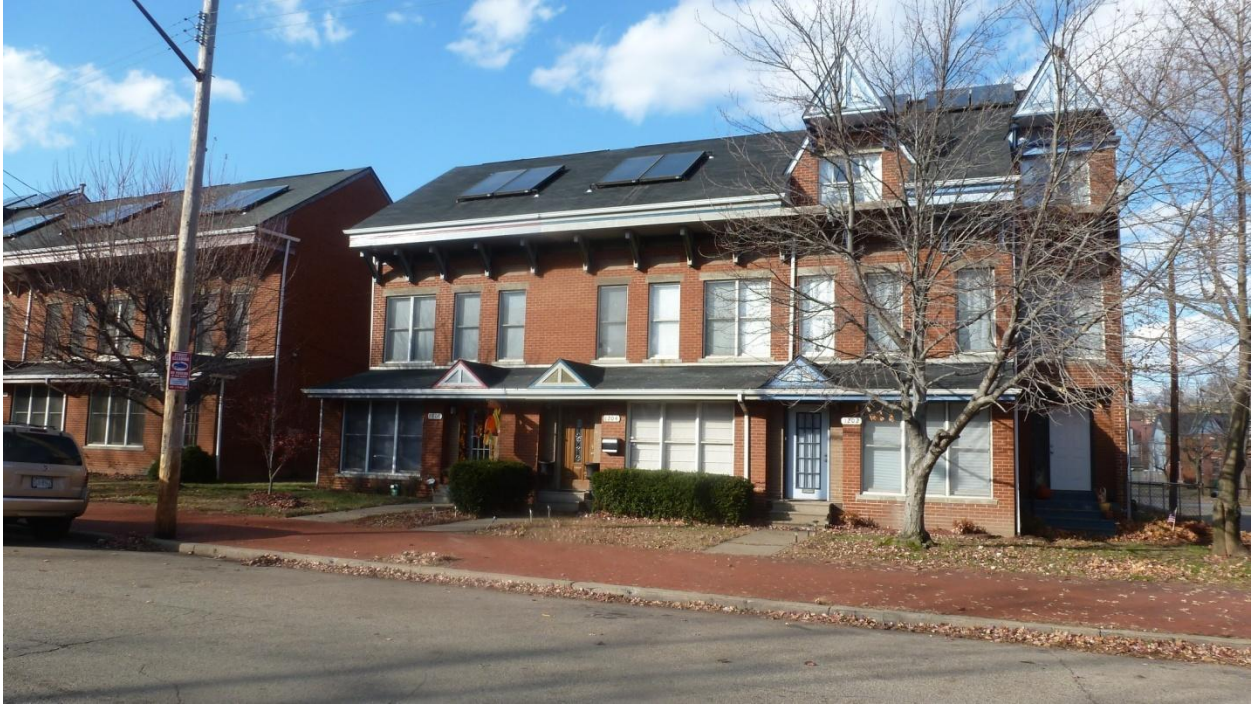
Pictures of 1300 th Block of Manchester as on November 14, 2014
