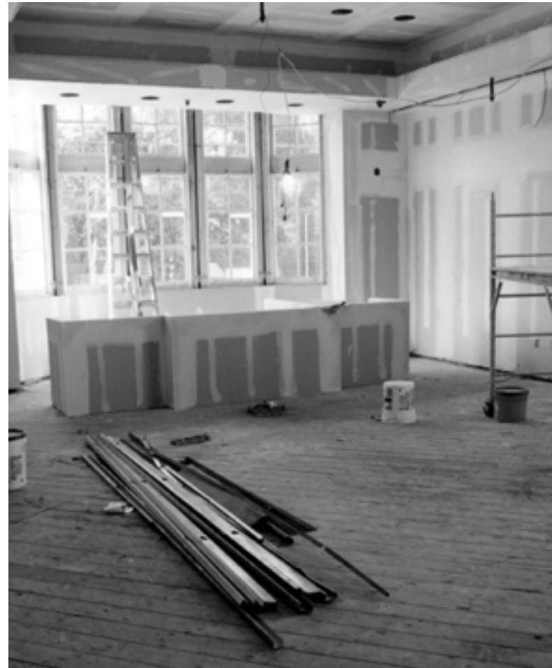
Justice Center construction
