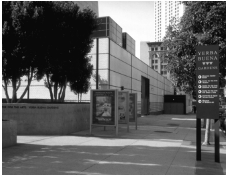
The Third Street facade of James Polshak's Center for the Arts has been criticized for the blank wall it presents to the street.
