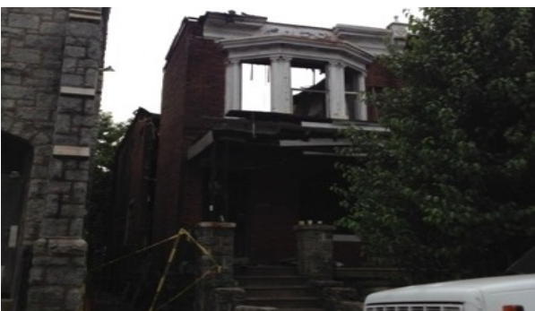
BEFORE - Sample abandoned home in neighborhood
