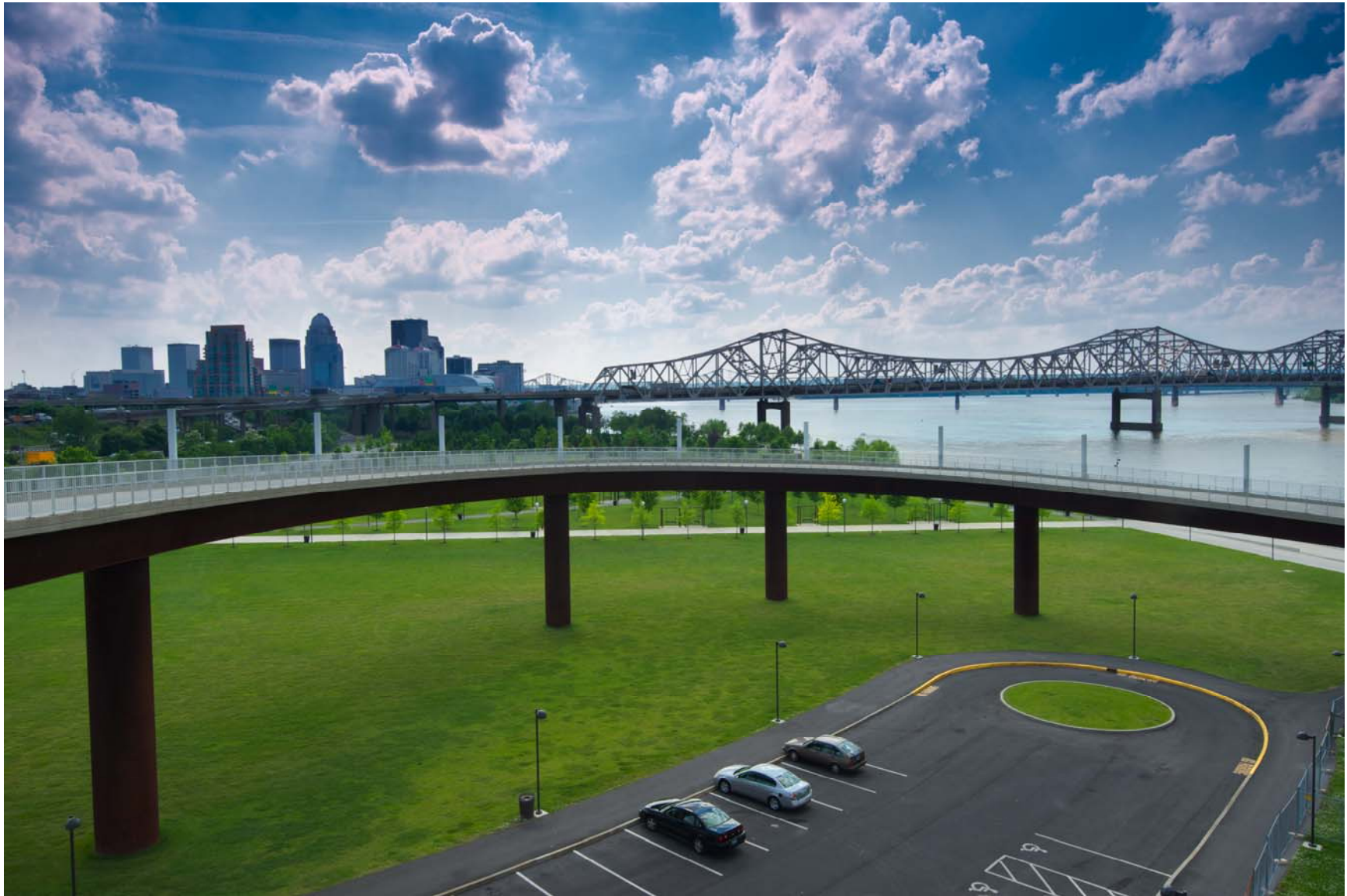
View of Waterfront Park from the ramp to the Big Four Bridge. The ramp is an unusual feat of engineering, curving back upon itself to spiral up to the bridge.
