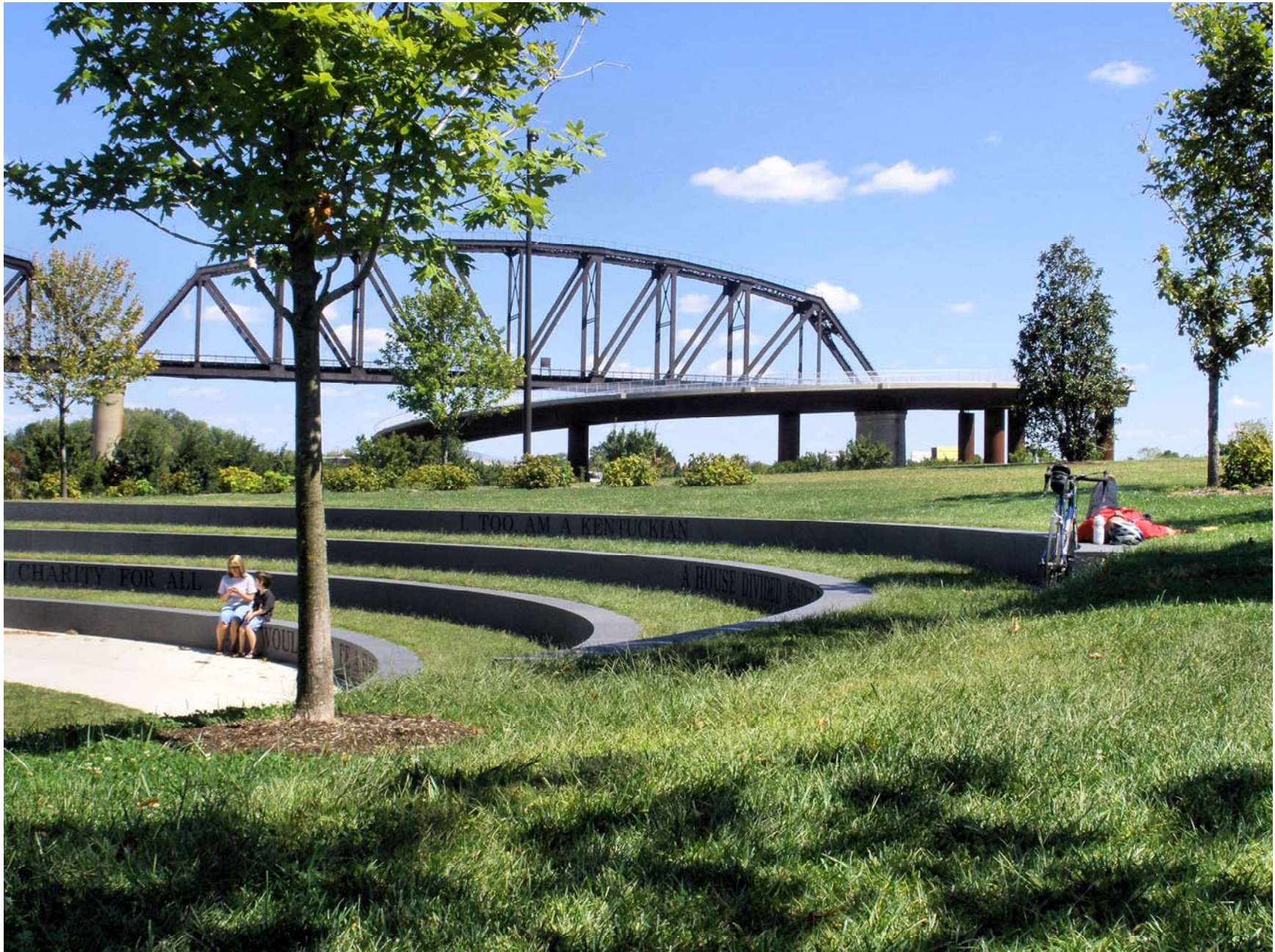
The Lincoln Memorial with the Big Four Pedestrian/Bicycle Bridge in the background.
